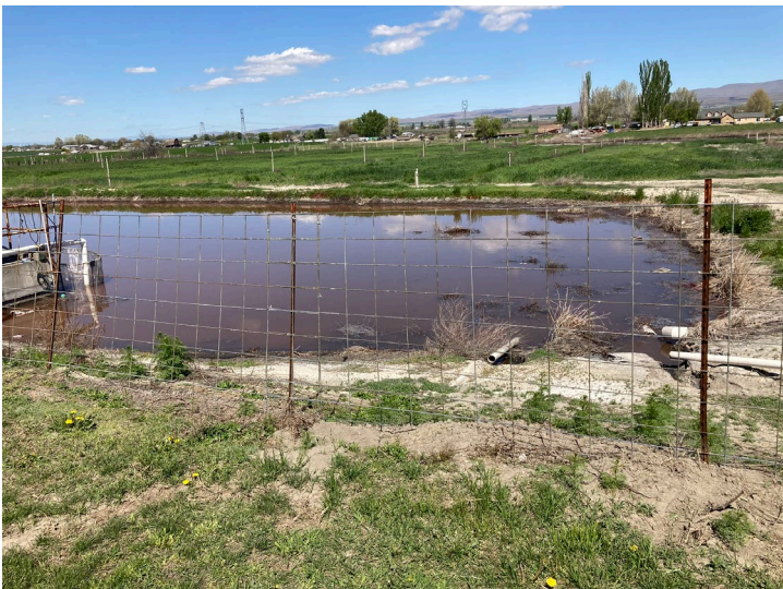
Photo 3 [IMG_0384] Description: Unlined wastewater lagoon that contains brine water and stormwater also diluted with irrigation water
