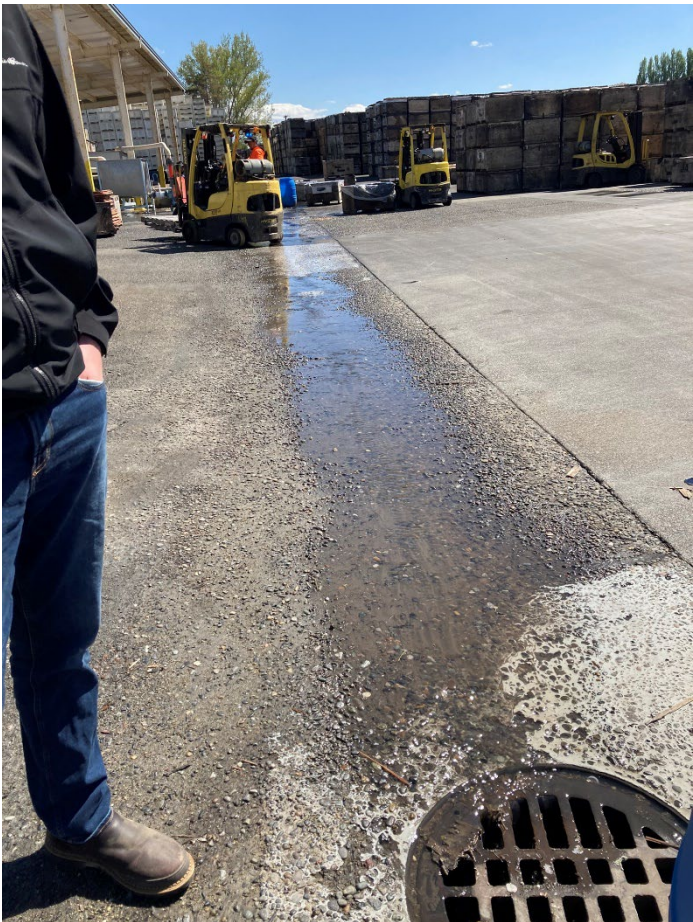
Photo 2 [IMG_0382] Description: Drain that collects stormwater and process water from sizer – goes to the lagoon
