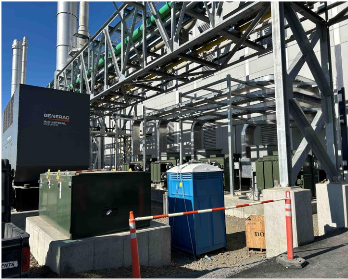
Figure 3: Generators and transformers on the right with secondary containment
