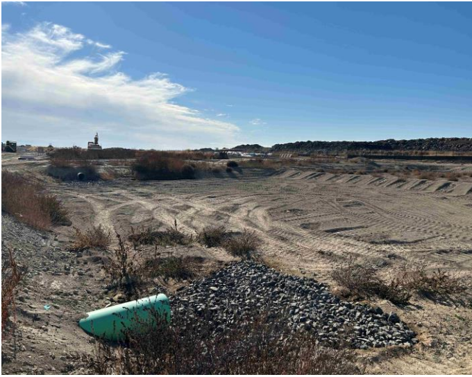
Figure 5: Stormwater infiltration pond with an outlet
