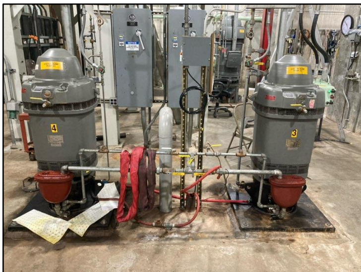
Figure 4- Station sump pumps 1 and 2 for discharge RR20
