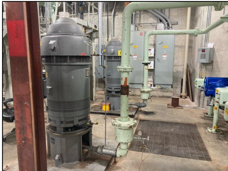
Figure 3- Unwatering sump pumps 1 and 2 for discharges RR18 and RR19
