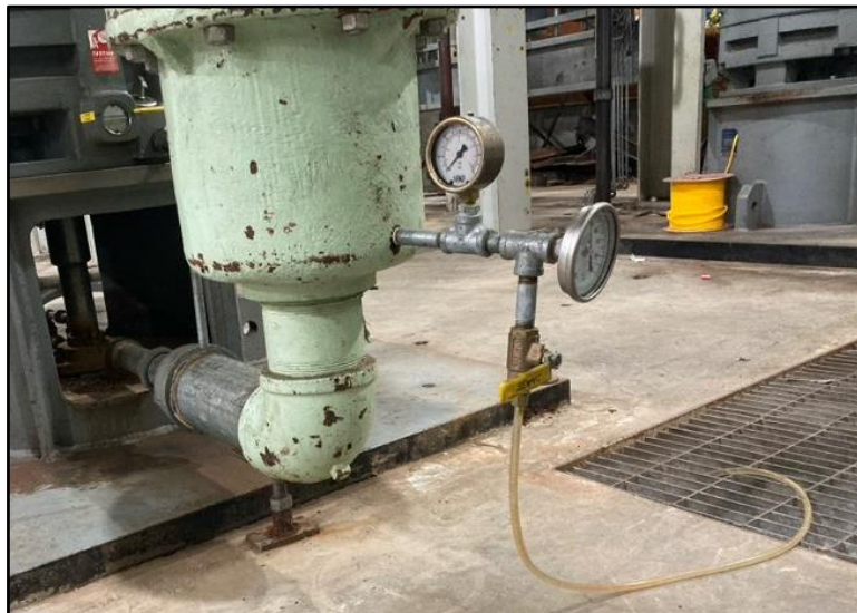
Figure 5- Oil and grease sample port for discharge RR18/RR19
