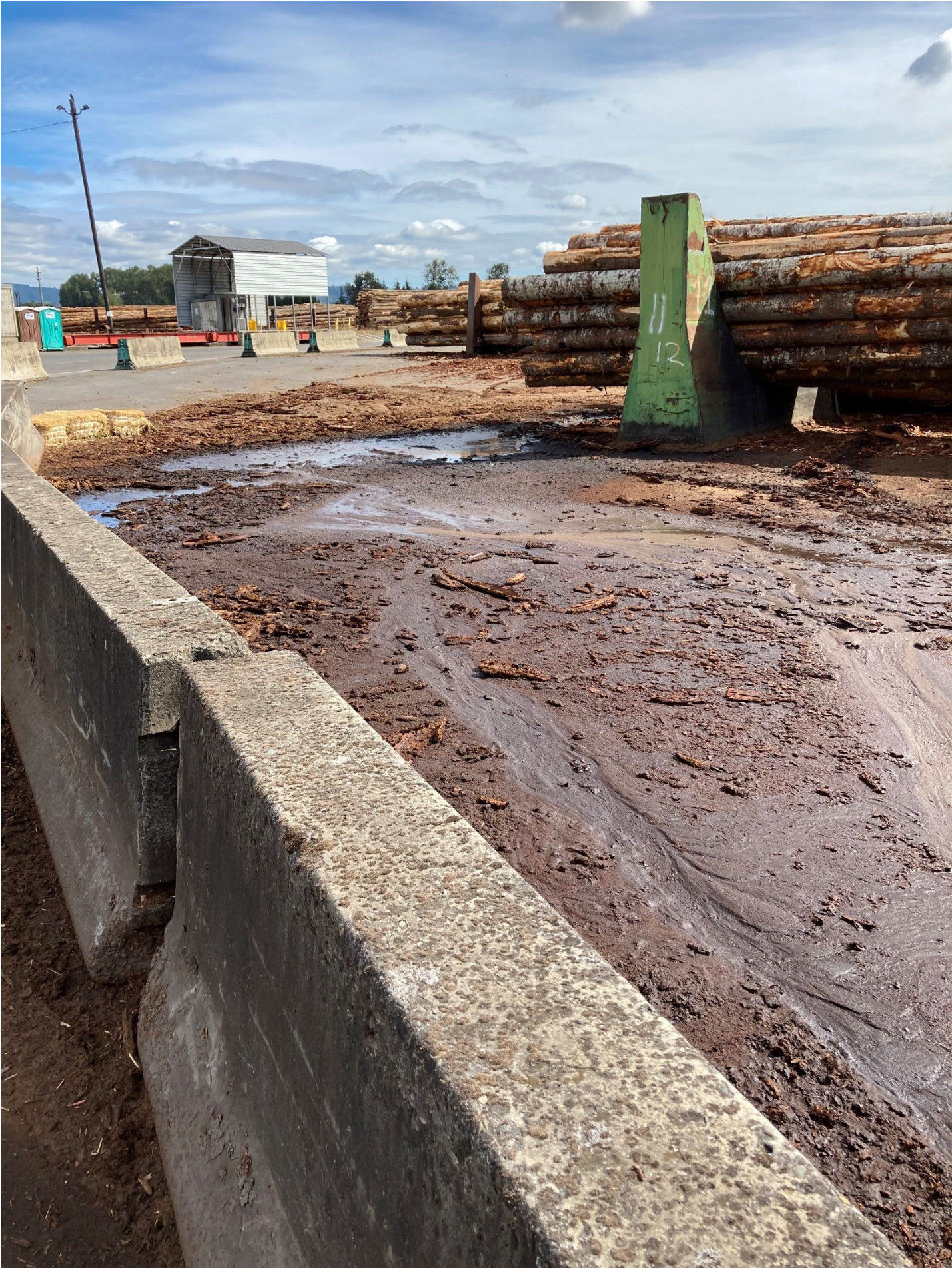
Photo 14: Wood fines and bark accumulated before jersey barriers near the discharge to NDP’s Chips Scale Sump.
