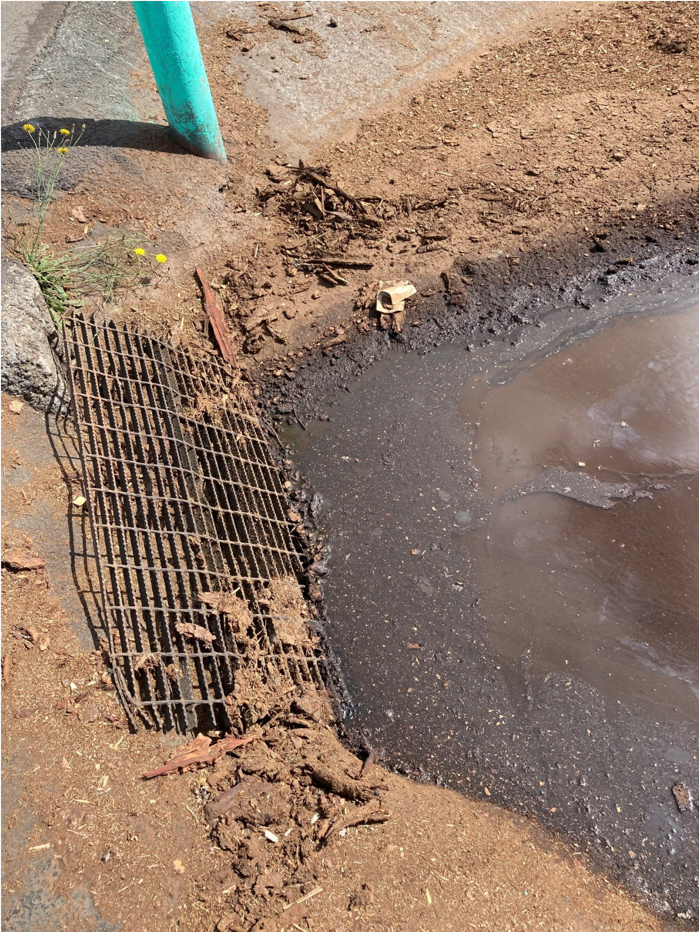
Photo 15: Bar screen at Weyerhaeuser’s discharge to NDP’s Chips Scale Sump.
