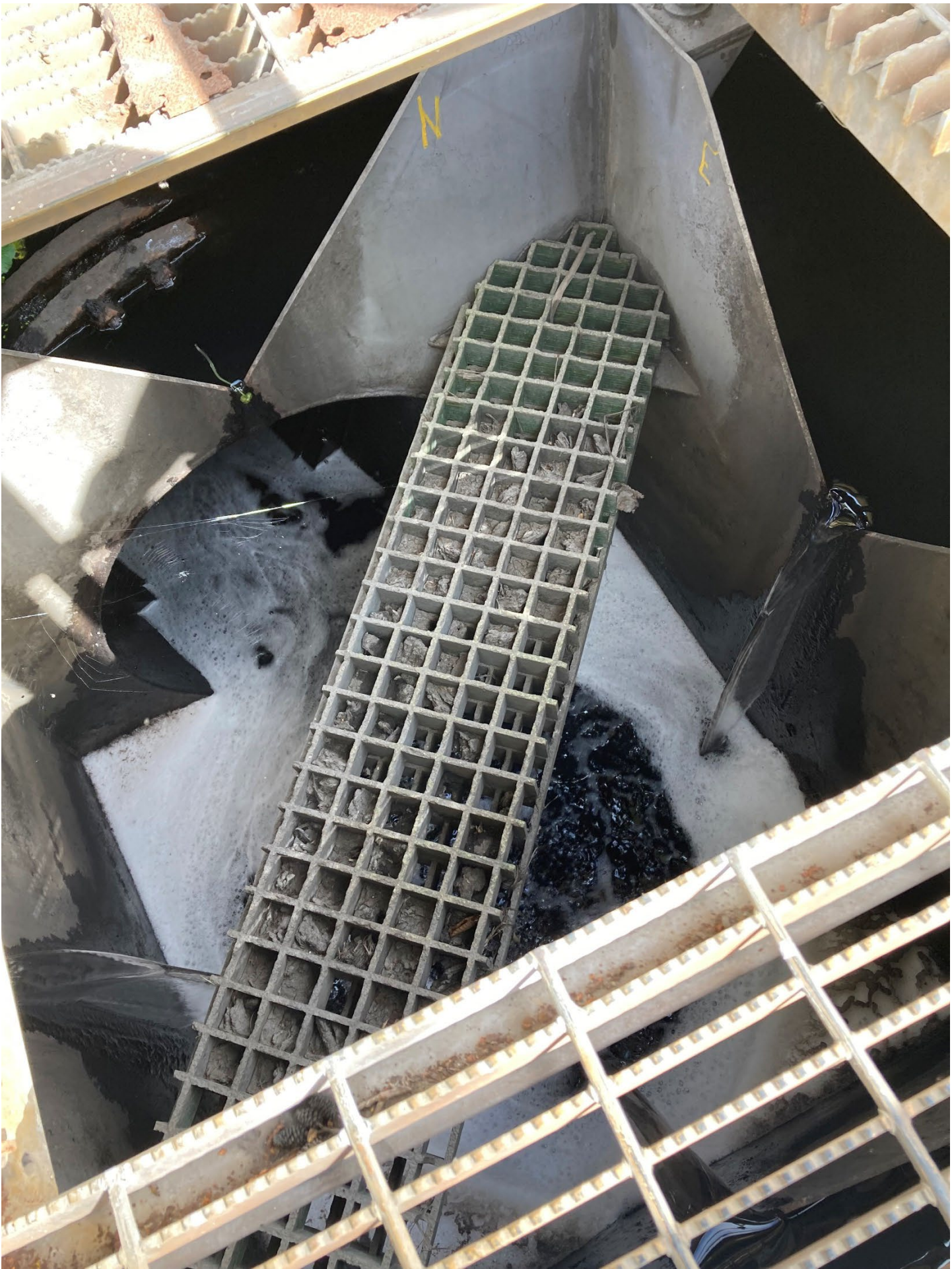
Photo 28: Outfall 003B discharge to CDID Ditch #3 and effluent weirs.
