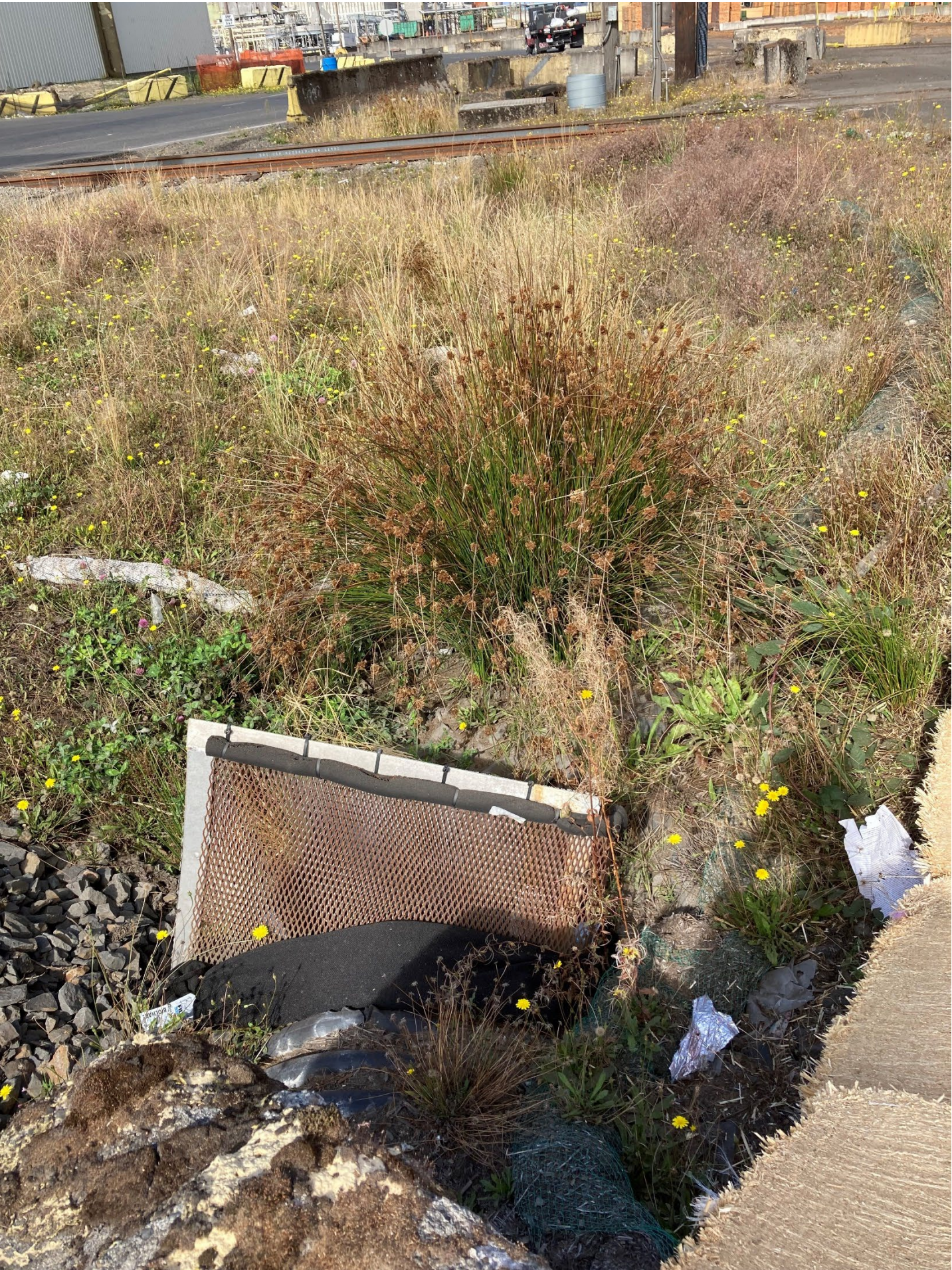
Photo 35: Stormwater culvert screen and drainage ditch in the Pipe A drainage basin.
