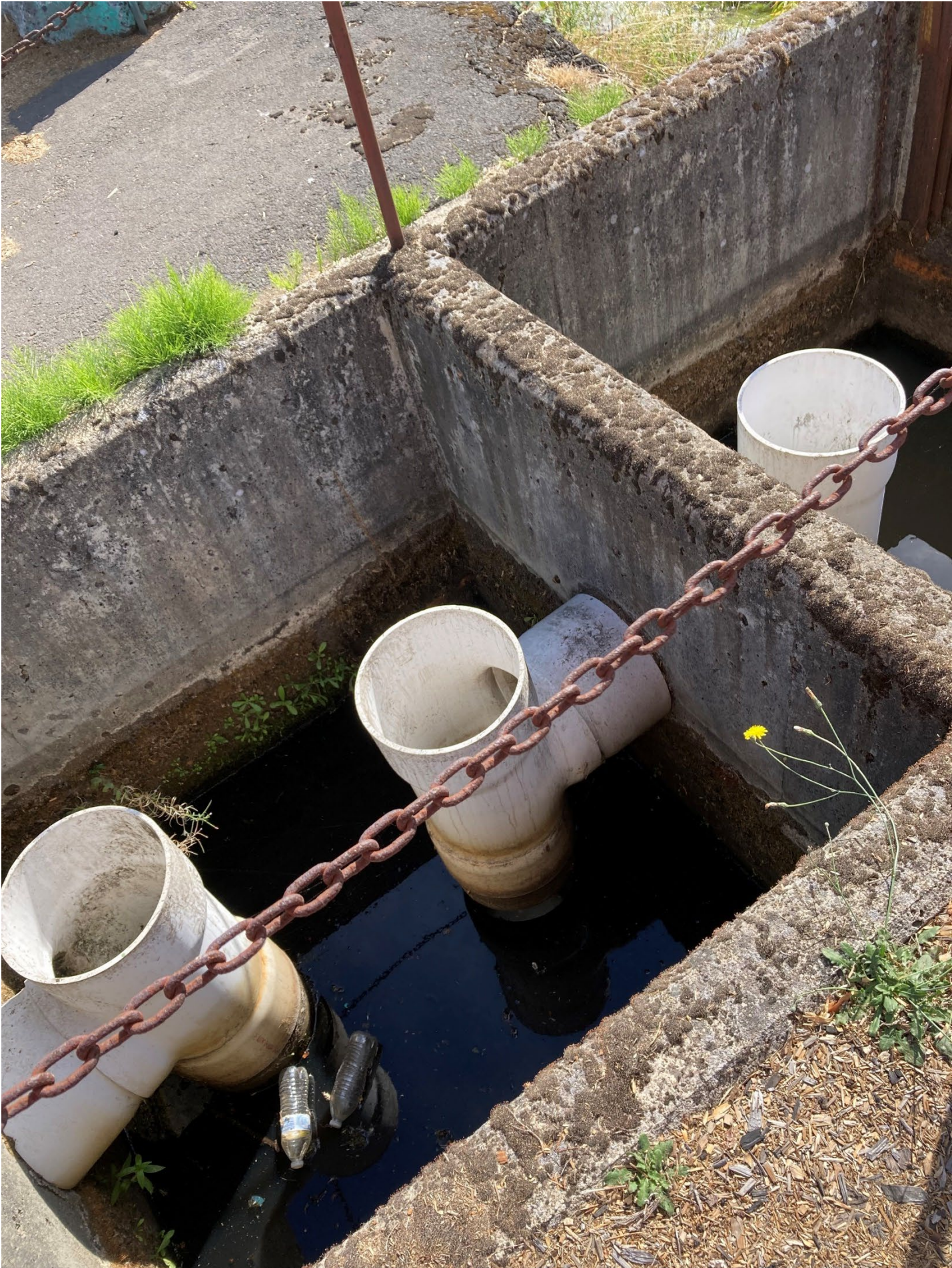
Photo 10: Old oil-water separator near the Stacker Shop and NDP’s chips area.
