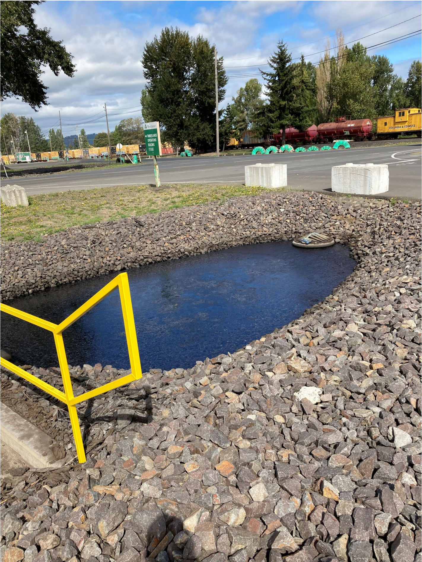
Photo 7: Conveyance ditch outlet downstream of the check dam located west of the TOB.
