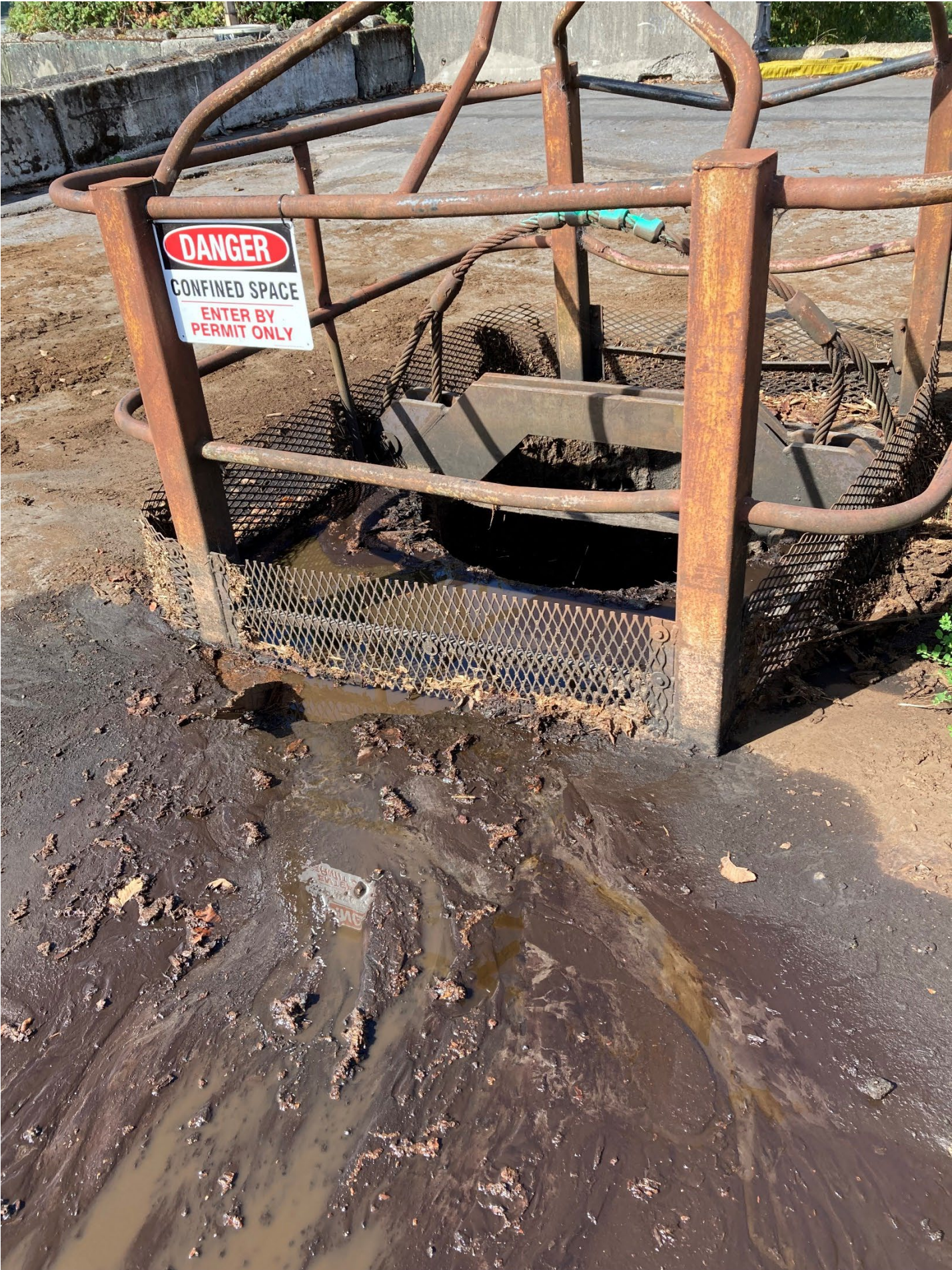
Photo 19: Runoff entering the Export Dock Sump.
