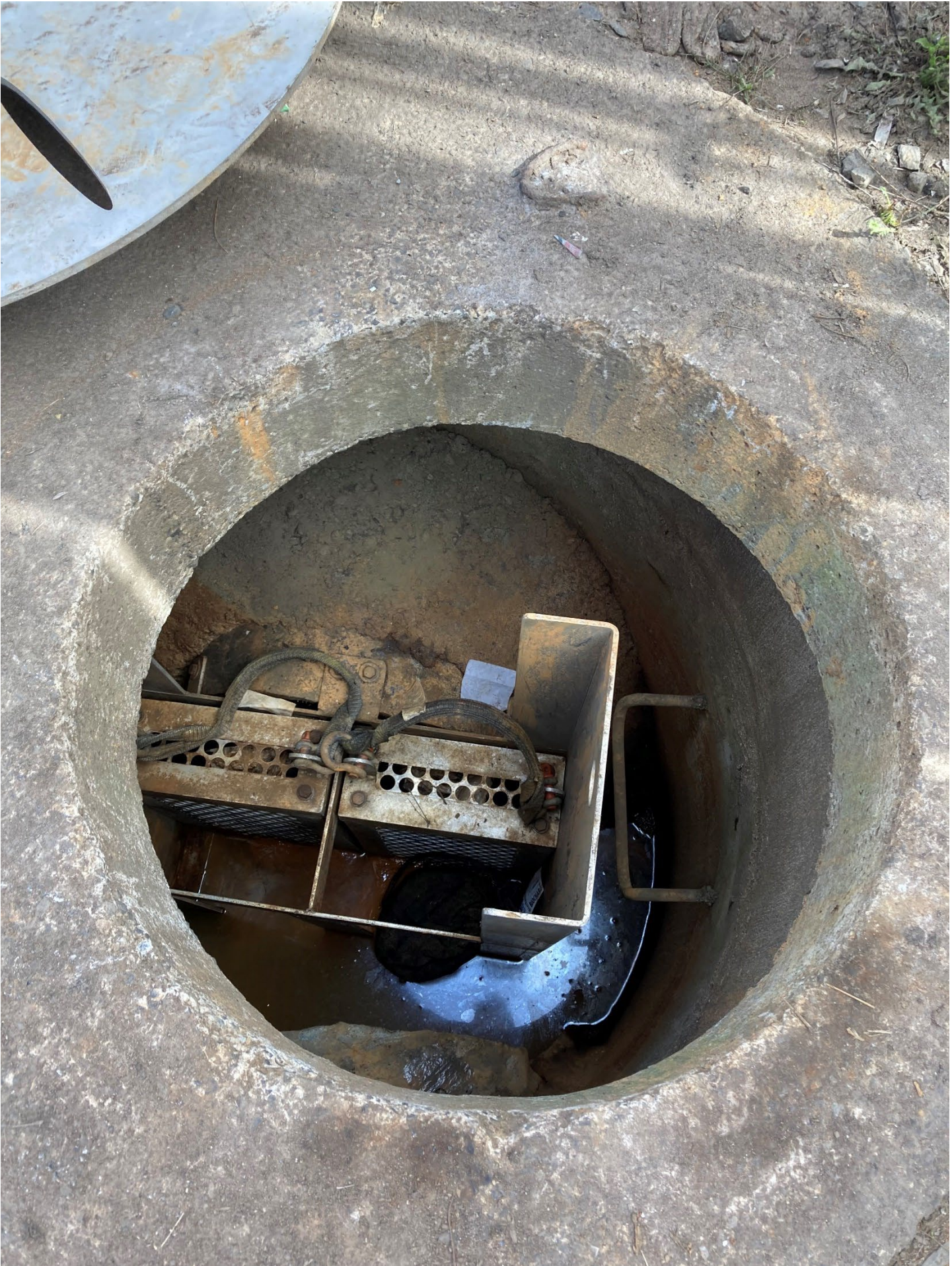
Photo 31: Manhole catch basin filtration structure in the Pipe A drainage area.
