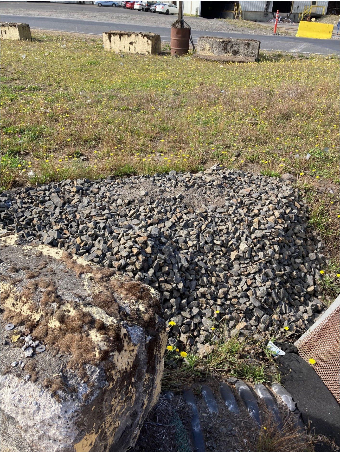
Photo 34: Rock installed near a stormwater drainage ditch in the Pipe A drainage basin.
