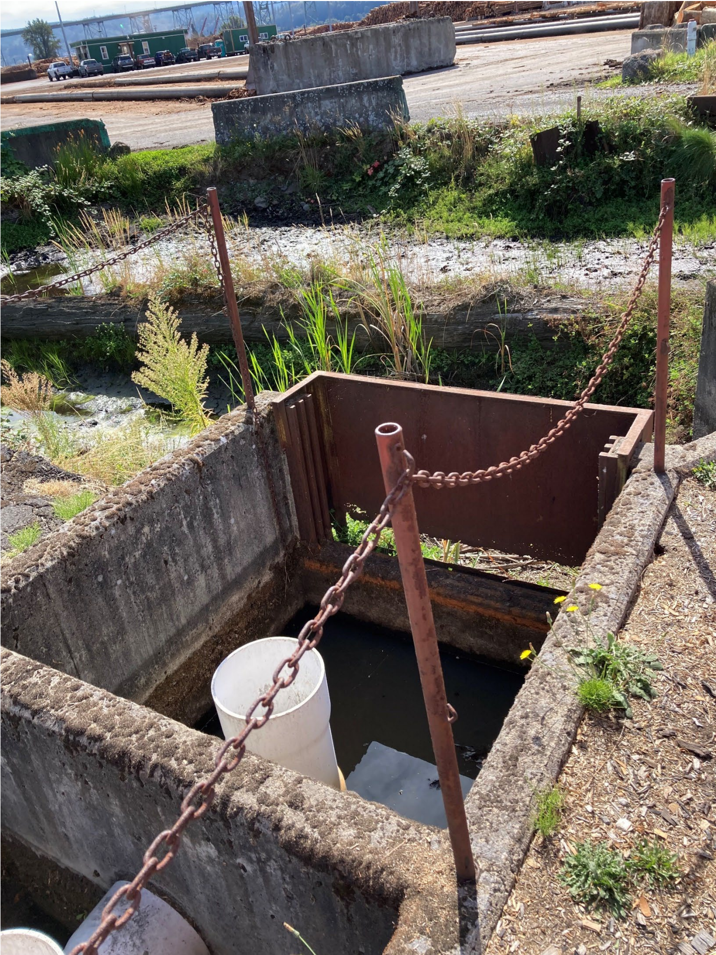
Photo 11: Old oil-water separator inlet near the Stacker Shop and NDP’s chips area.
