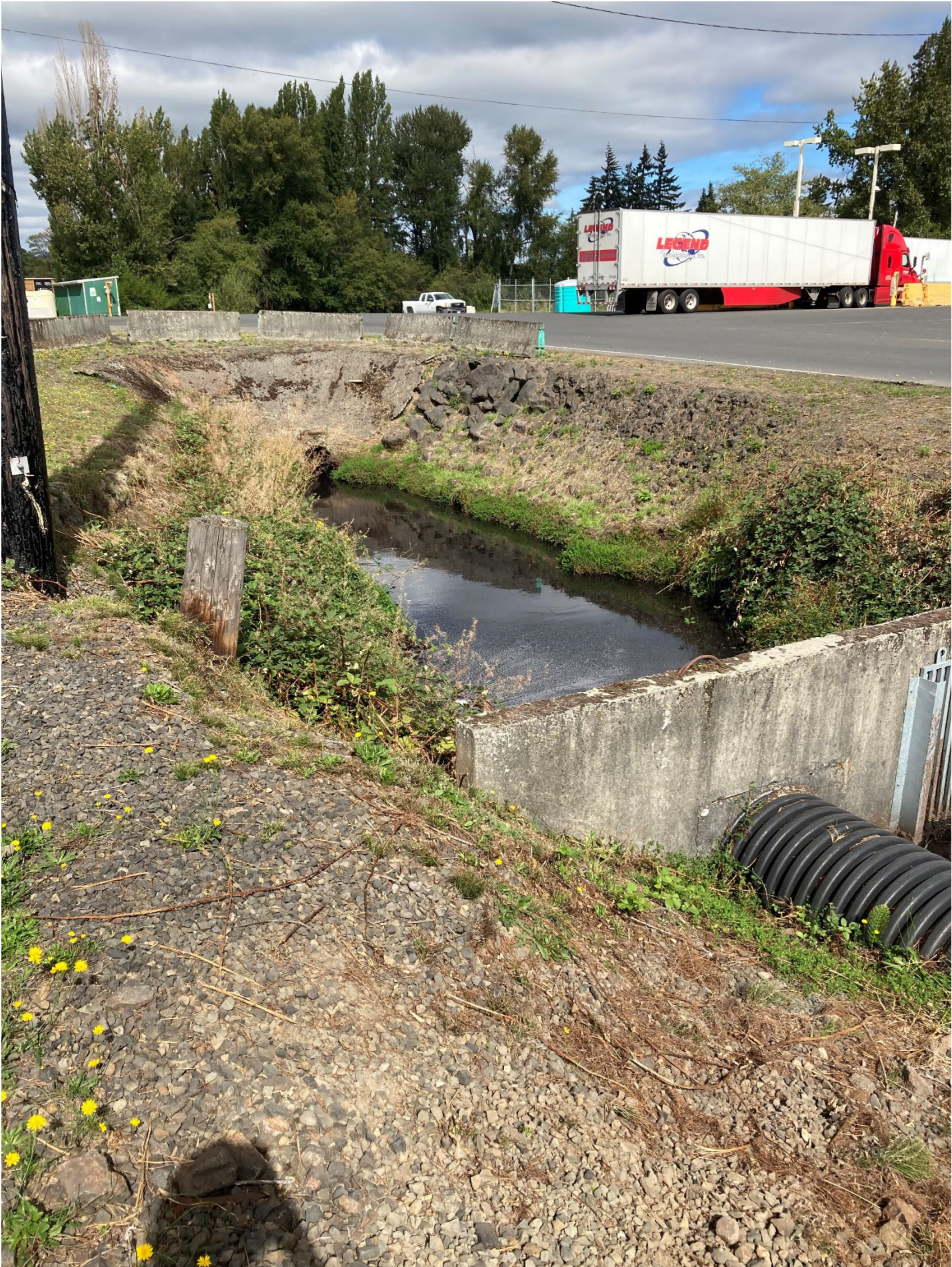
Photo 4: Conveyance ditch downstream of bar screen and inlet of East Sump, Export Dock pump, and eastern conveyance ditches.
