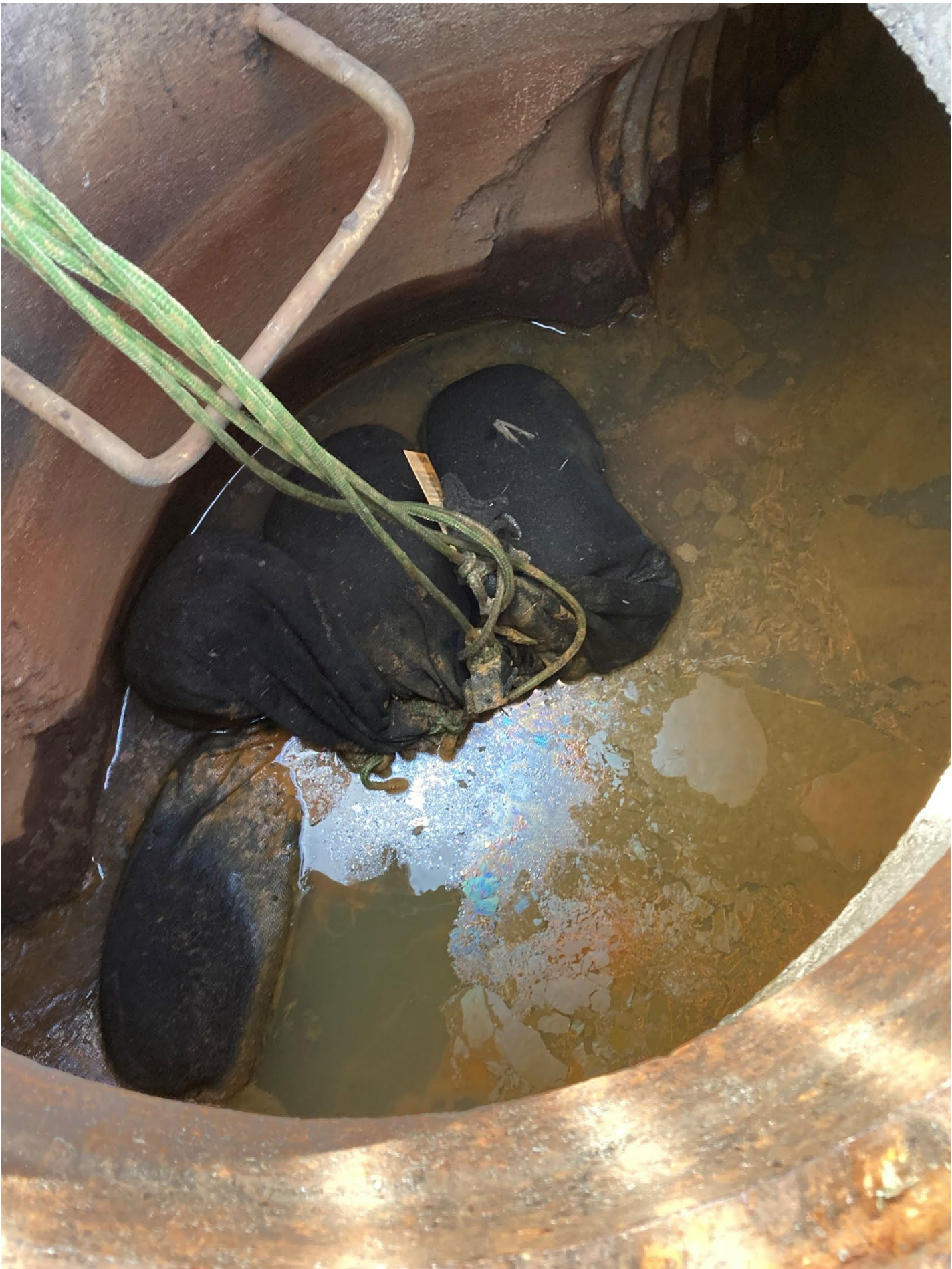
Photo 33: Biochar bags in a manhole catch basin in the Pipe A drainage area.
