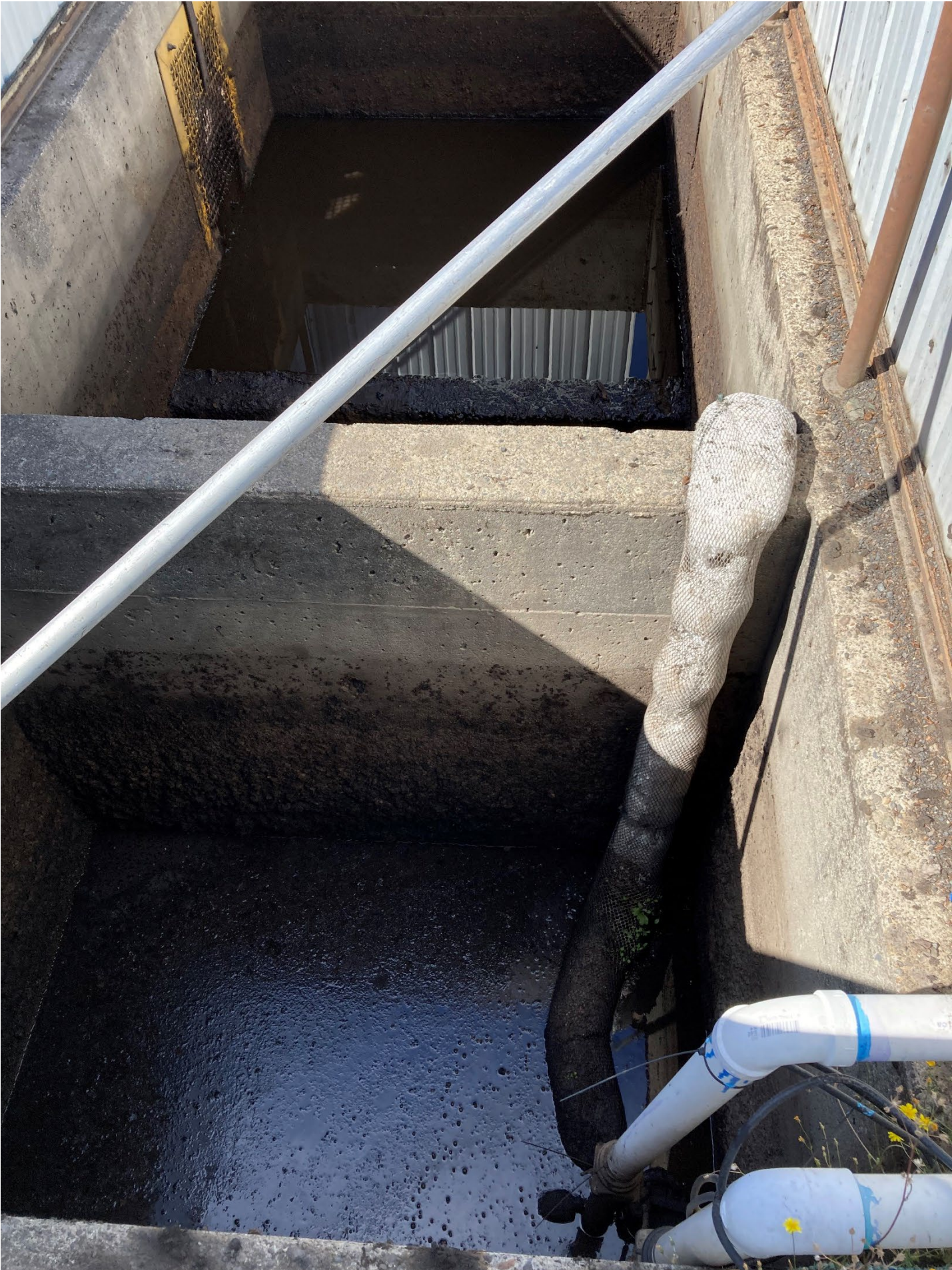
Photo 9: Scum and solids in the sump where Outfall 001B pumps to NDP’s Industrial WWTP.
