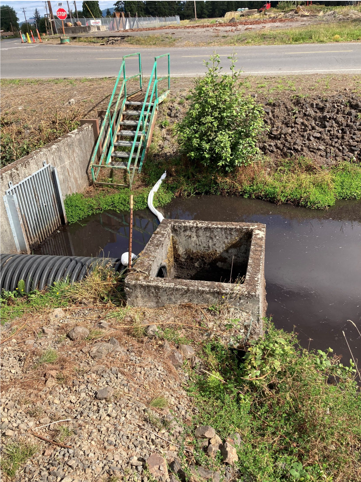
Photo 3: Inlet and bar screen at the conveyance ditch receiving the East Sump and eastern conveyance ditches runoff.
