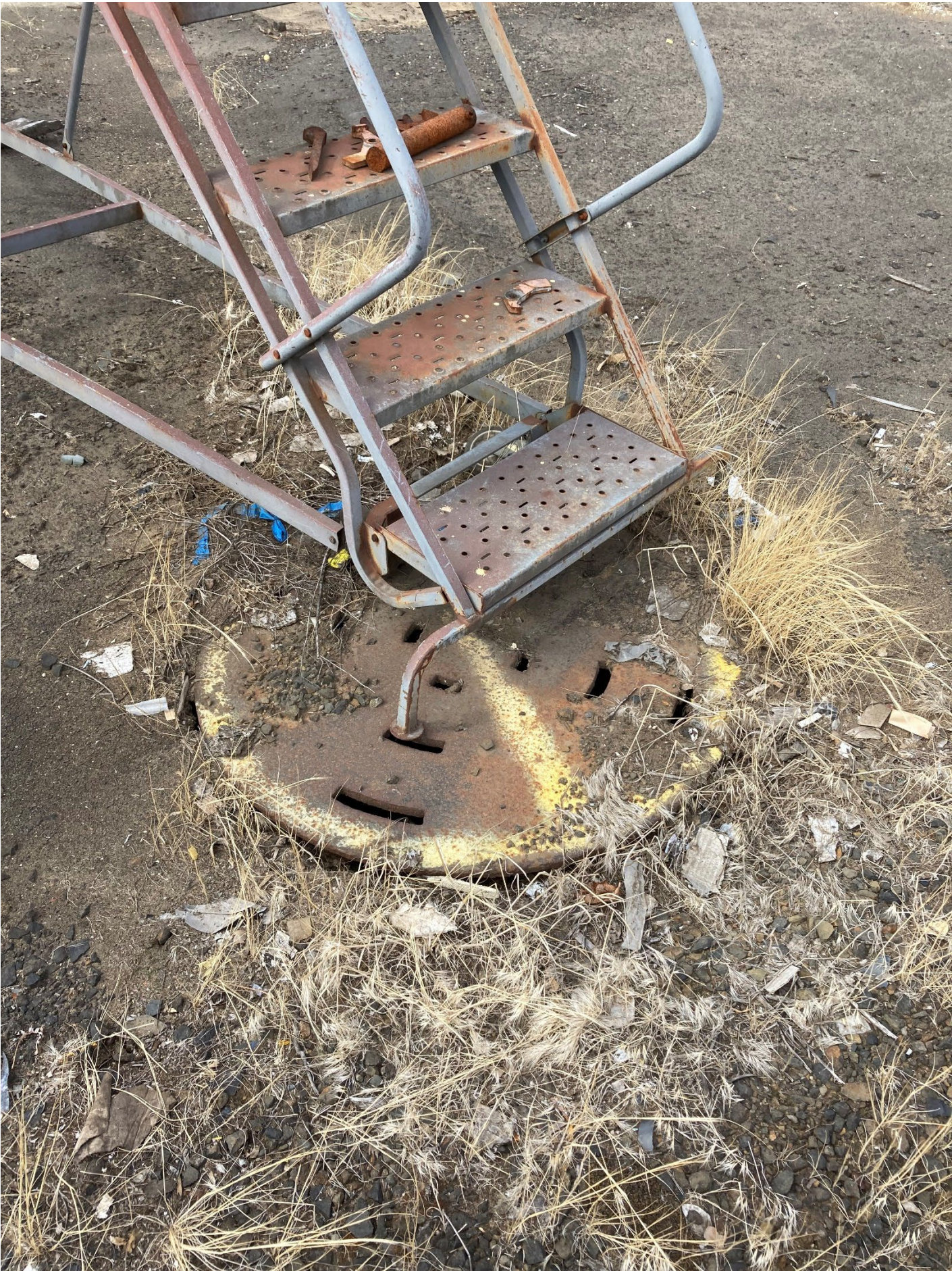
Photo 38: Stormwater catch basin on the neighboring CLC property apparently within the Pipe N drainage basin.
