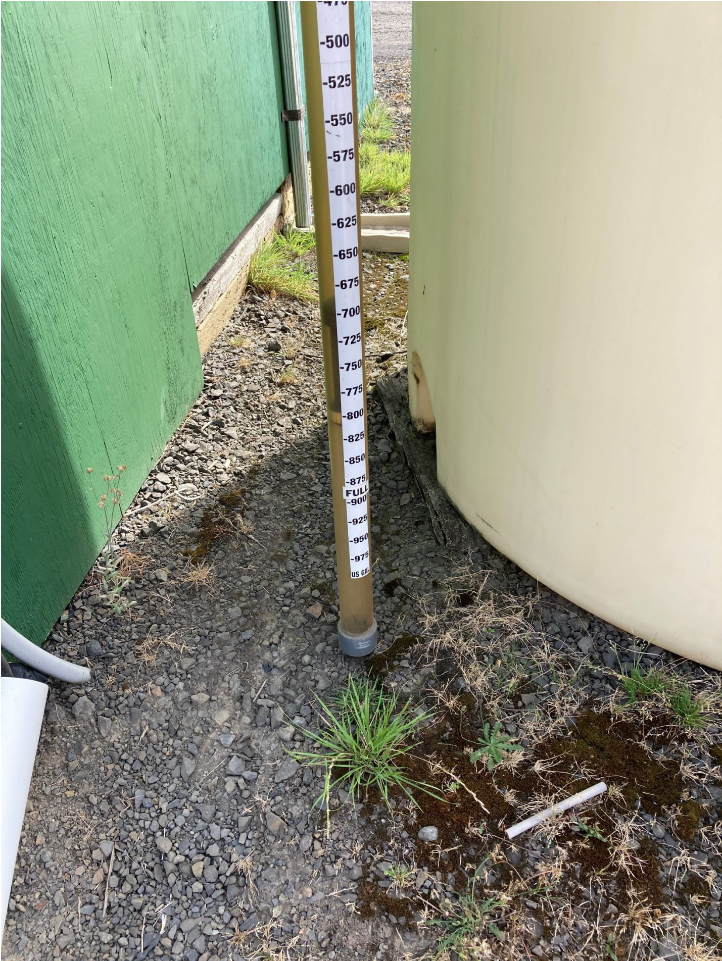
Photo 26: Sodium hydroxide tank level indicator.
