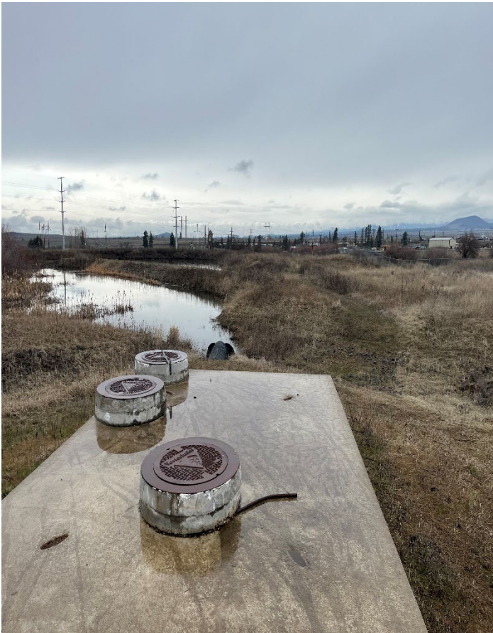
Photo 4 [IMG_0480] Description: Stormwater pond and pretreatment vaults.
