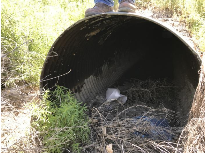
FIGURE 11 FIRST CULVERT IS ALSO SLOWLY FILLING WITH SEDIMENT.
