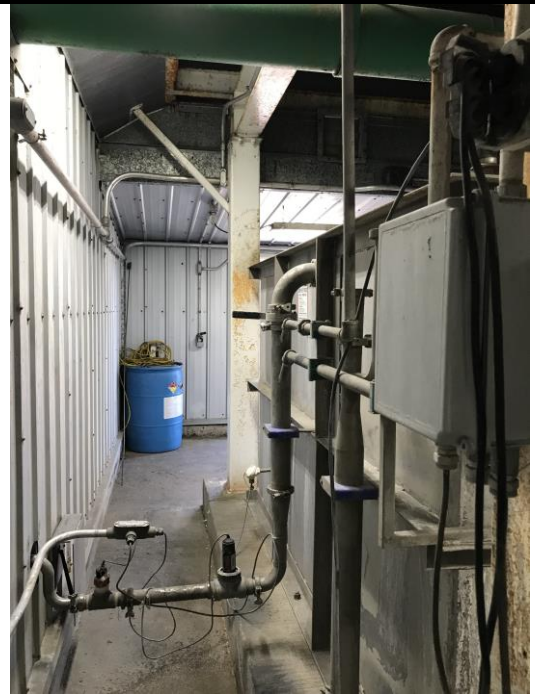
FIGURE 12 NON-CONTACT COOLING WATER PH AND TEMPERATURE METERS
