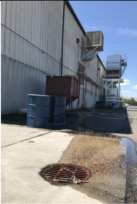
FIGURE 7 COOLING UNITS CONDENSATE DRAINS TO SUMP FIRST FLUSH SYSTEM.
