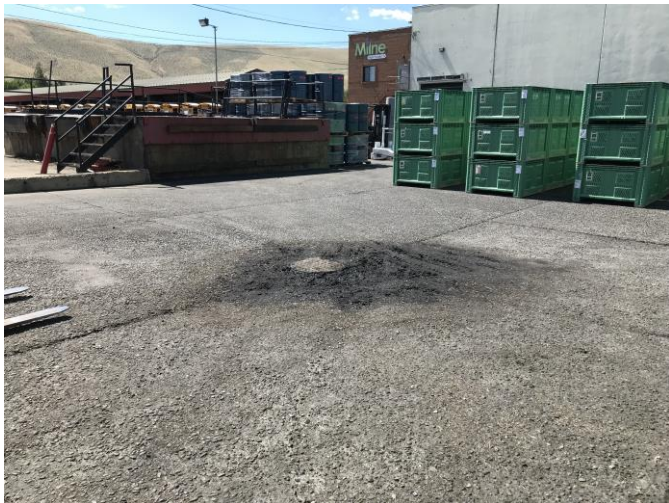
FIGURE 3: NORTH SIDE DRAIN ON ACID PITTED CONCRETE FROM FRUIT JUICES. DRAINS TO SANITARY SEWER
