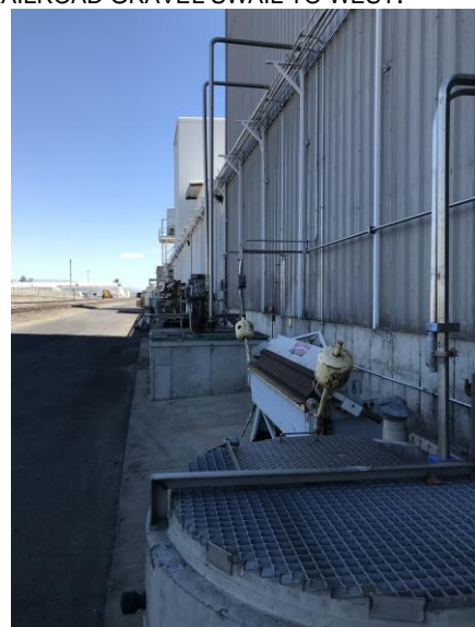
FIGURE 6: ALMOST ENTIRE WEST SIDE OF FACILITY DRAINS TO THIS SUMP PUMP "FIRST FLUSH" SYSTEM, WHICH IS ROUTED TO POTW
