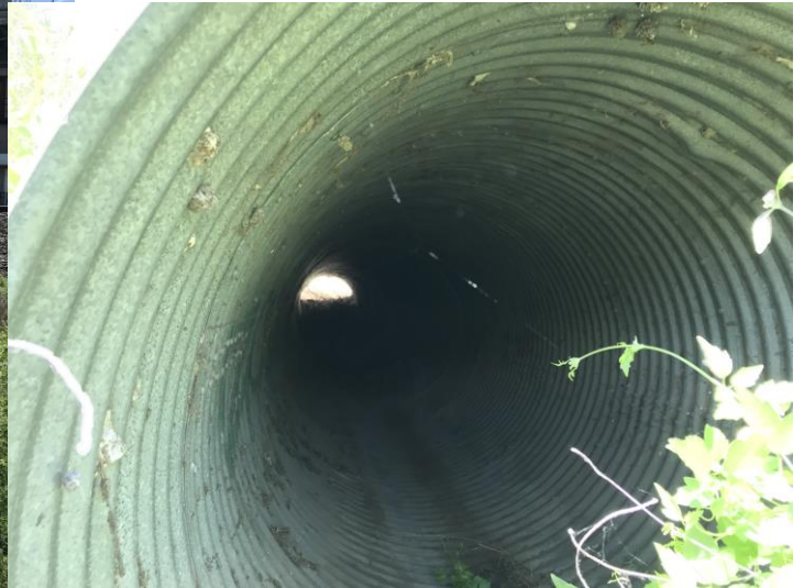
FIGURE 10 SEDIMENT HAS FILLED IN THIS CULVERT'S FINAL OUTFALL HALFWAY. END OF CULVERT IS TO BE DESIGNATED AS THE COMPLIANCE SAMPLING POINT.
