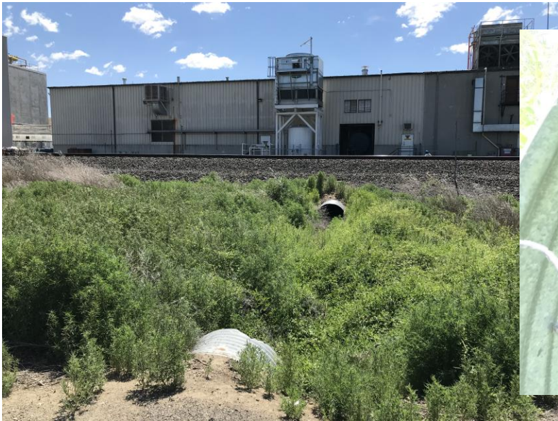
FIGURE 9 CULVERTS LEAD TO YAKIMA RIVER
