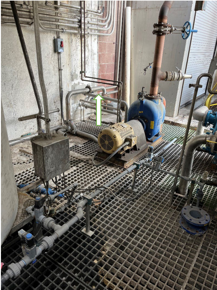
Photo 1 [IMG_0617] Description: Grated sewer vault that stores wastewater going to the city POTW. The pipe indicated allows cooling water to discharge to outfall 001.
