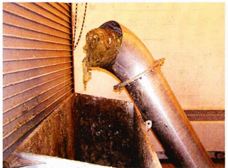
PHOTO #:03 DATE: 10/18/05, 10:36 AM FILE: SMITH/PA180020.JPG TAKEN BY: JARON SMITH DESCRIPTION: INFLUENT SCREENINGS DISPOSAL.
