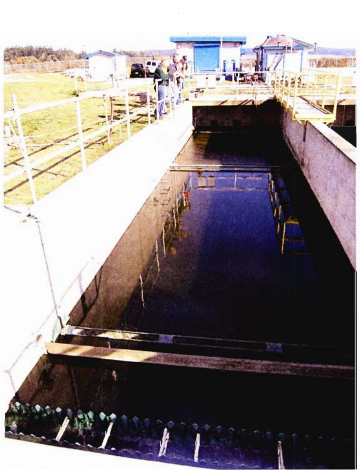
PHOTO #028 DATE: 10/18/05, 2:36 PM FILE: MCKONE/PA180046.JPG TAKEN BY: SHAWN MCKONE DESCRIPTION: LAGOON TERTIARY TREATMENT BASIN FOR ALGAE REMOVAL.
