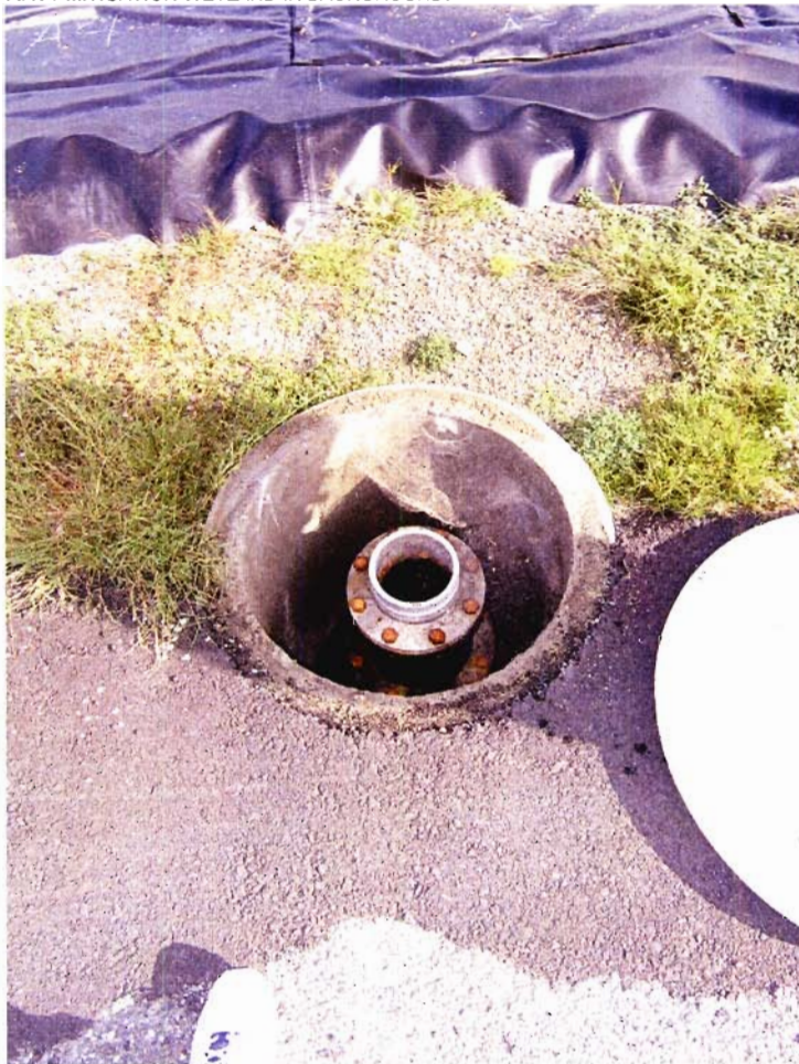
PHOTO #027 DATE: 10/18/05, 2:17 PM FILE: MCKONE/PA180039.JPG TAKEN BY: SHAWN MCKONE DESCRIPTION: EXTRACTION PORT FOR ANAEROBIC LAGOON SOLIDS REMOVAL..
