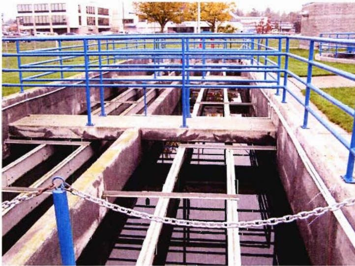
PHOTO #:015 DATE: 10/18/05, 10:22 AM FILE: SMITH/PA180016.JPG TAKEN BY: JARON SMITH DESCRIPTION: CHLORINE CONTACT CHAMBERS.
