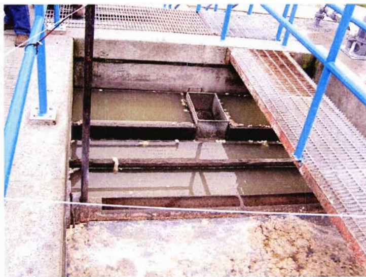
PHOTO #09 DATE: 10/18/05, 11:11 AM FILE: SMITH/PA180035.JPG TAKEN BY: JARON SMITH DESCRIPTION: PRIMARY SEDIMENTATION BASIN, EFFLUENT END.
