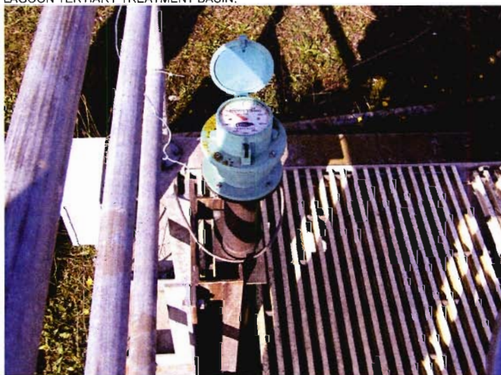
PHOTO #:031 DATE: 10/18/05, 2:36 PM FILE: SMITH/PA180074.JPG TAKEN BY: JARON SMITH DESCRIPTION: EFFLUENT FLOW METER, PROPELLER TYPE, AT LAGOON TERTIARY TREATMENT AREA.
