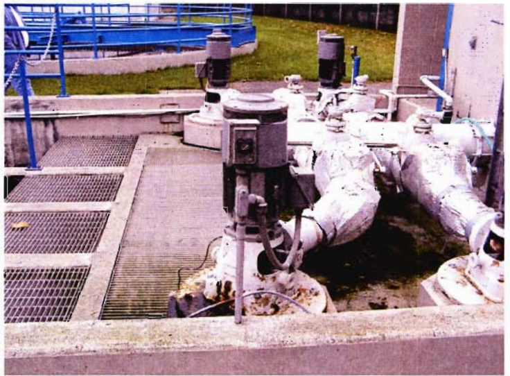
PHOTO #:016 DATE: 10/18/05, 11:32 AM FILE: SMITH/PA180053.JPG TAKEN BY: JARON SMITH DESCRIPTION: FINAL EFFLUENT DISCHARGE PUMPS. USED ONLY AT HIGH TIDES WHEN EFFLUENT IS NOT ABLE TO PROPERLY FLOW UNDER GRAVITY.
