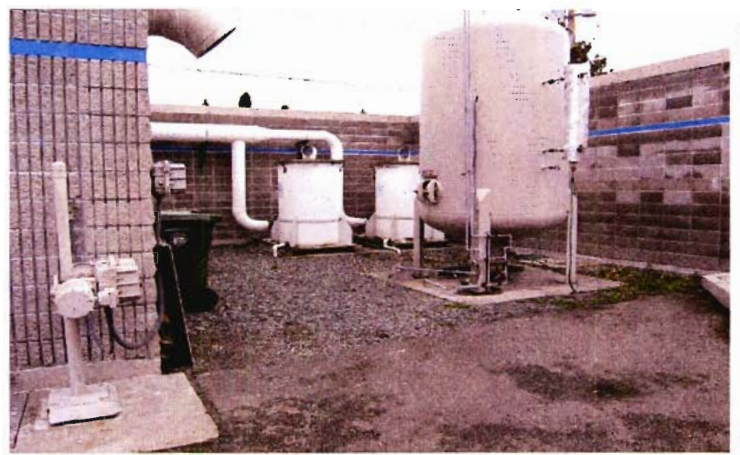
PHOTO #:05 DATE: 10/18/05, 10:45 AM FILE: MCKONE/PA180011.JPG TAKEN BY: SHAWN MCKONE DESCRIPTION: SURGE TANK AND CARBON ODOR SCRUBBERS OUTSIDE OF DIVERSION PUMP STATION
