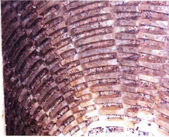
PHOTO #:013 DATE: 10/18/05, 11:18 AM FILE: MCKONE/PA180027.JPG TAKEN BY: SHAWN MCKONE DESCRIPTION: EFFLUENT END RBC DISCS, END VIEW.
