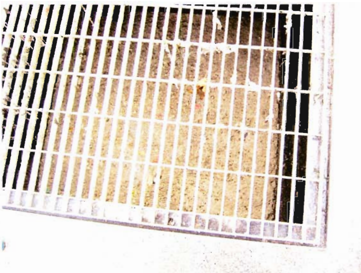
PHOTO #08 DATE: 10/18/05, 11:00 AM FILE: MCKONE/PA180018.JPG TAKEN BY: SHAWN MCKONE DESCRIPTION: COLLECTED SCUM IN SCUM BASIN. COLLECTED SCUM IS PUMPED TO DIGESTERS ON A WEEKLY BASIS
