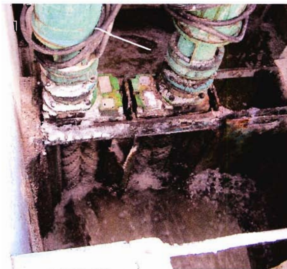
PHOTO #:024 DATE: 10/18/05, 2:04 PM FILE: SMITH/PA180063.JPG TAKEN BY: JARON SMITH DESCRIPTION: MACERATORS AT LAGOON HEADWORKS.
