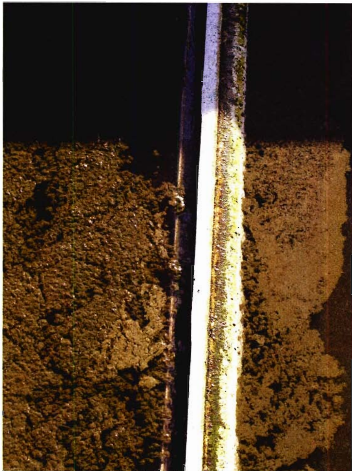
PHOTO #:029 DATE: 10/18/05, 2:37 PM FILE: McKONE/PA180047.JPG TAKEN BY: SHAWN MCKONE DESCRIPTION: COAGULATED ALGAE BEING SKIMMED FROM THE SURFACE OF THE LAGOON TERTIARY TREATMENT BASIN.
