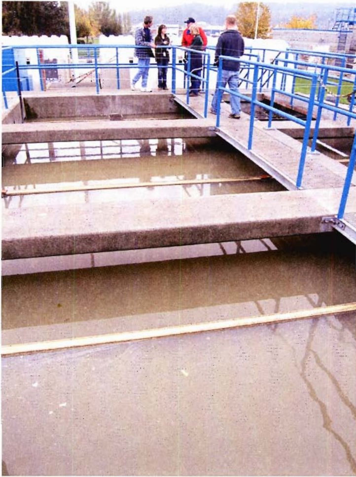
PHOTO #:010 DATE: 10/18/05, 11:06 AM FILE: MCKONE/PA180021.JPG TAKEN BY: SHAWN MCKONE DESCRIPTION: PRIMARY SEDIMENTATION BASINS.
