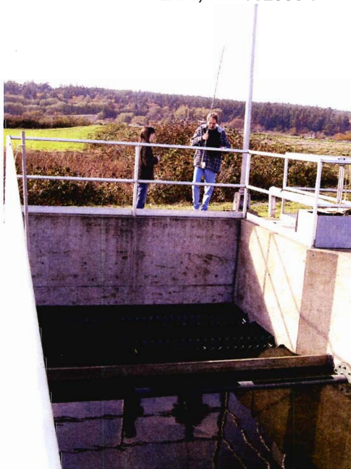
PHOTO #:030 DATE: 10/18/05, 2:56 PM FILE: McKONE/PA180050.JPG TAKEN BY: SHAWN MCKONE DESCRIPTION: GRAB SAMPLING FOR CHLORINE RESIDUAL AT THE DISCHARGE END OF THE LAGOON TERTIARY TREATMENT BASIN.
