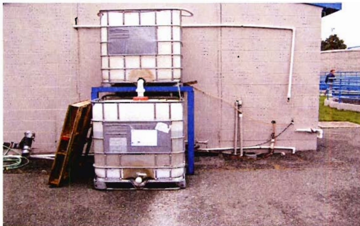
PHOTO #:04 DATE: 10/18/05, 10:24 AM FILE: SMITH/PA180018.JPG TAKEN BY: JARON SMITH DESCRIPTION: CHEMICAL (COAGULANT) STORAGE NEAR SECONDARY CLARIFIERS.
