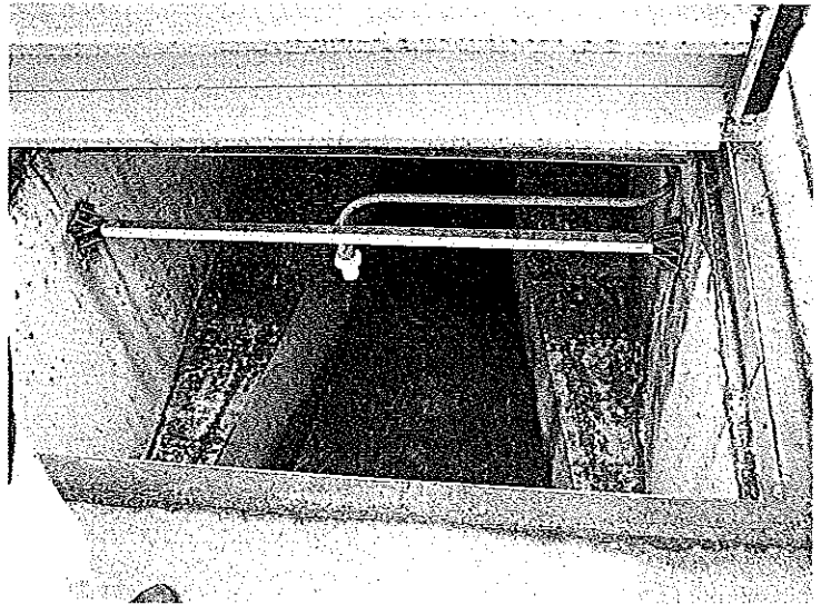
PHOTO #:10 DATE: 12/05/06 TAKEN BY: GREG STEGMAN FILE NO.:PC050015.JPG DESCRIPTION: PRIMARY FLOW METER/FLUME
