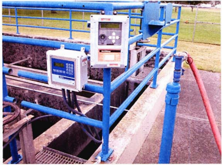
04 DATE: 6/28/2007 TAKEN BY: McKONE FILE No.: OH062007_9 TIME: 10:43AM DESCRIPTION: FLOW METER LOCATION AT THE HEAD OF THE CHLORINE CONTACT CHAMBER. NEW CONTROL UNIT (ON THE LEFT, OLD UNIT ON THE RIGHT.
