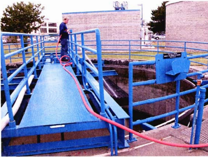
PHOTO #:05 DATE: 6/28/2007 TAKEN BY: McKONE FILE No.: OH062007_7 TIME: 10:42AM DESCRIPTION: NORTH SECONDARY CLARIFIER IN THE PROCESS OF BEING CLEANED
