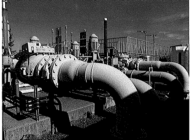
PHOTO #:06 DATE: 09/23/08 TAKEN BY: LAURA FRICKE DESCRIPTION: SAND FILTER PUMPING
