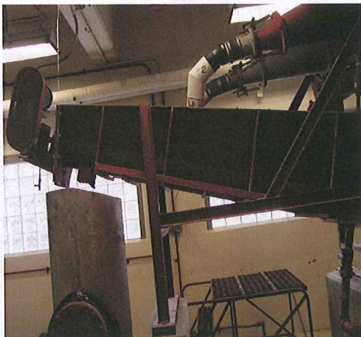
PHOTO #:05 DATE: 02/21/2012 TAKEN BY: MONIKA KANNADAGULI DESCRIPTION: INFLUENT BAR SCREEN BYPASS CHANNEL.
