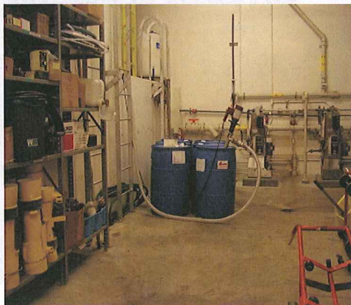
PHOTO #:12 DATE: 02/21/2012 TAKEN BY: MONIKA KANNADAGULI DESCRIPTION: POLYMER ADDED TO GRAVITY THICKENER.
