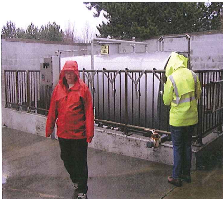
PHOTO #:15 DATE: 02/21/2012 TAKEN BY: MONIKA KANNADAGULI DESCRIPTION: DIESEL STORAGE FOR EMERGENCY GENERATOR.
