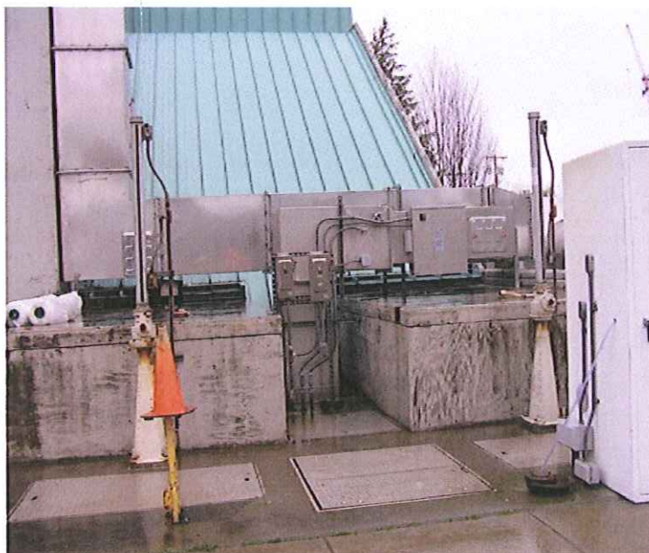
PHOTO #:03 DATE: 02/21/2012 TAKEN BY: MONIKA KANNADAGULI DESCRIPTION: SCREW PUMPS (UNDER METAL ROOF) LIFT INFLUENT INTO BAR SCREENS.
