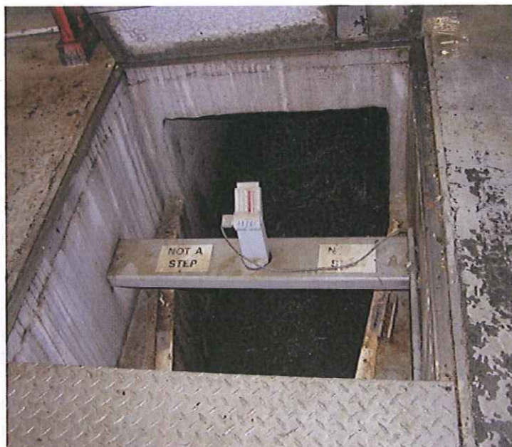
PHOTO #:06 DATE: 02/21/2012 TAKEN BY: MONIKA KANNADAGULI DESCRIPTION: FLOW MONITORING OVER THE INFLUENT CHANNEL.
