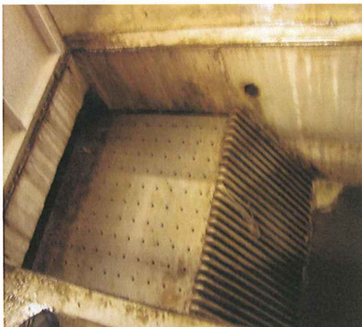
PHOTO #:05 DATE: 02/21/2012 TAKEN BY: MONIKA KANNADAGULI DESCRIPTION: INFLUENT BAR SCREEN BYPASS CHANNEL.
