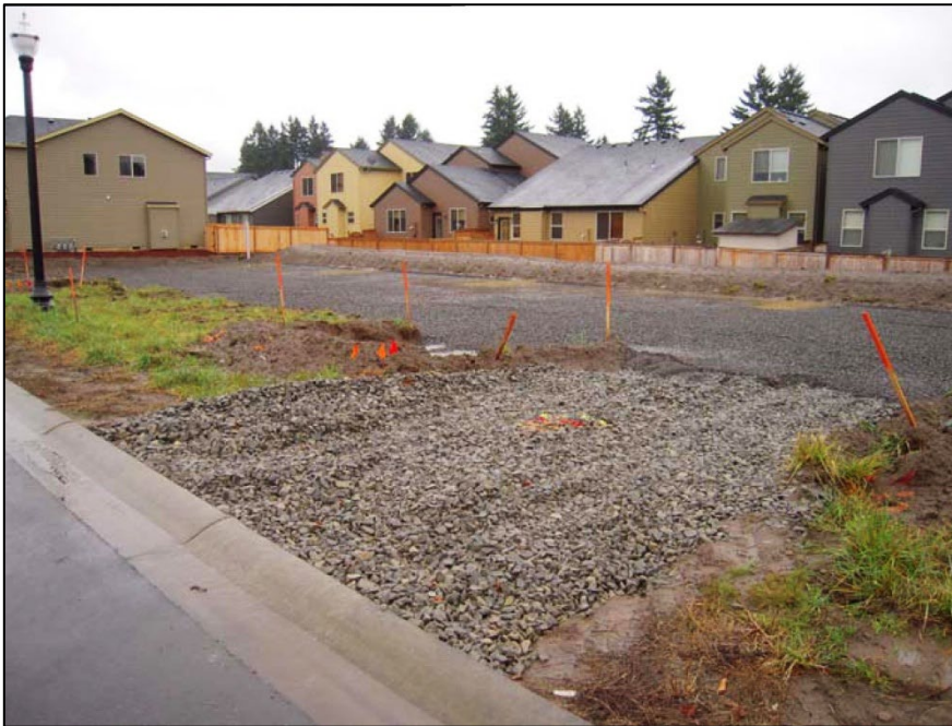
Figure 33: Small-scale Construction Entrance
