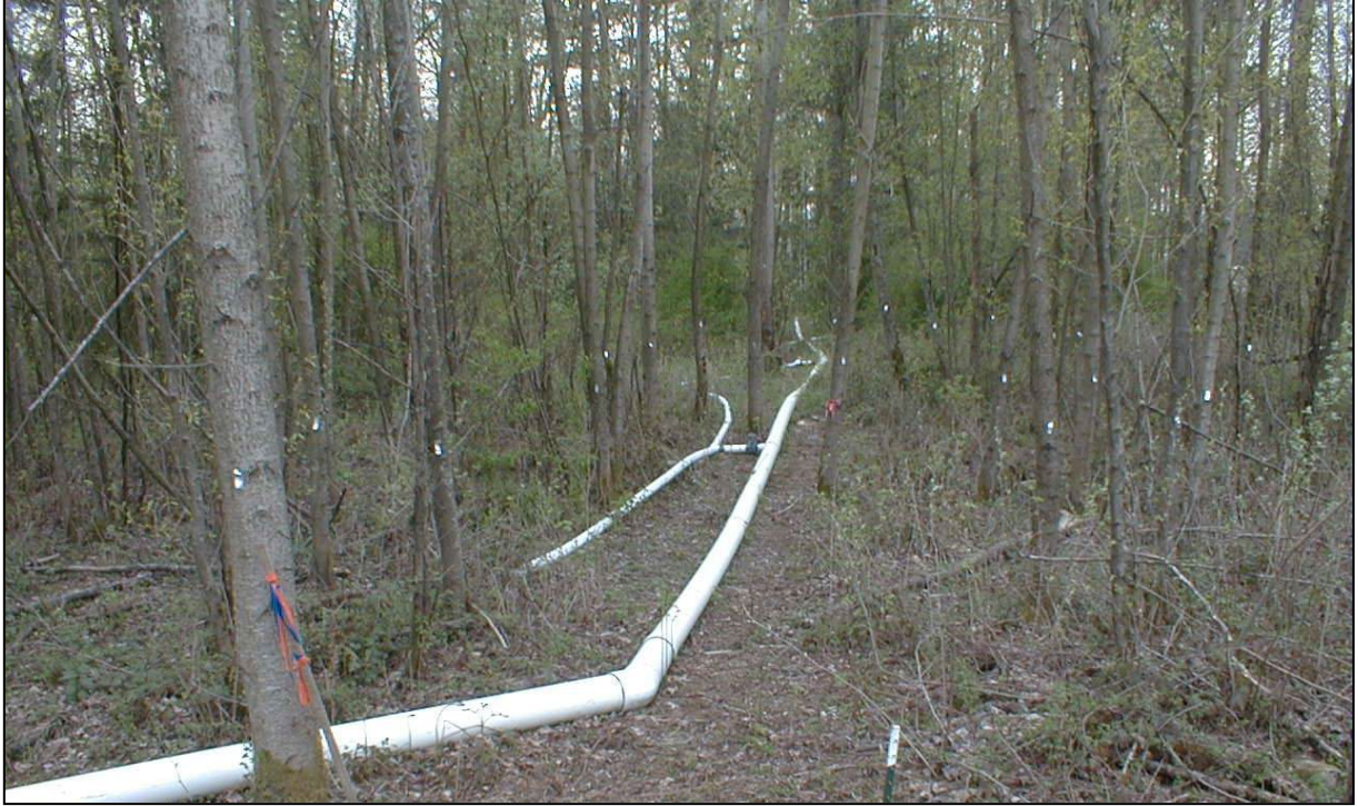
Figure 9.27: Manifold and Branches in a wooded, vegetated spray field
