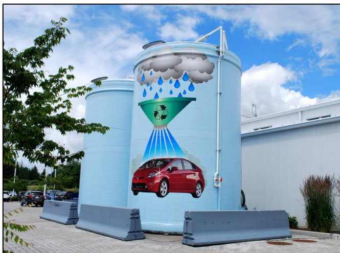
Figure 2.27: Cistern for Rainwater Harvesting
