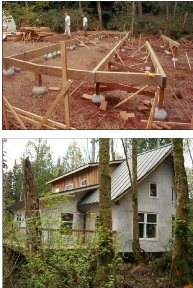
Figure 2.26: Pin Pier Foundation Construction & Completed Project, Bainbridge Island
