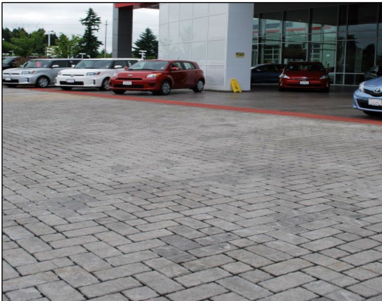
Figure 2.17: Permeable Pavement Application
