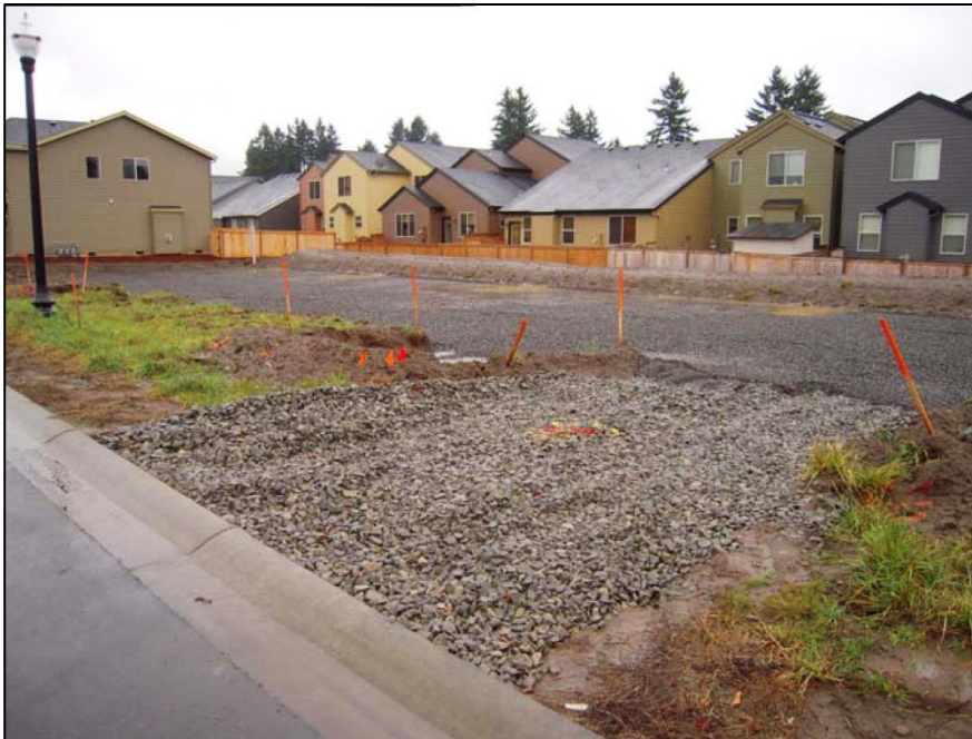
Figure 9.2: Small-scale Construction Entrance
