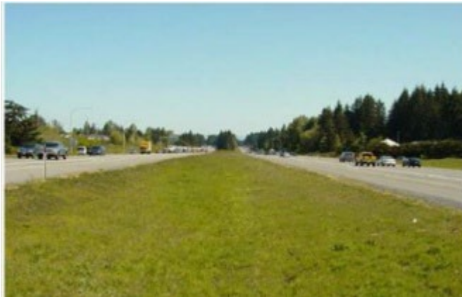
Figure 4.24: Compost-amended Vegetated Filter Strip Photo
