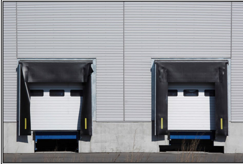
Figure 2.7: Loading Dock with Door Skirt
