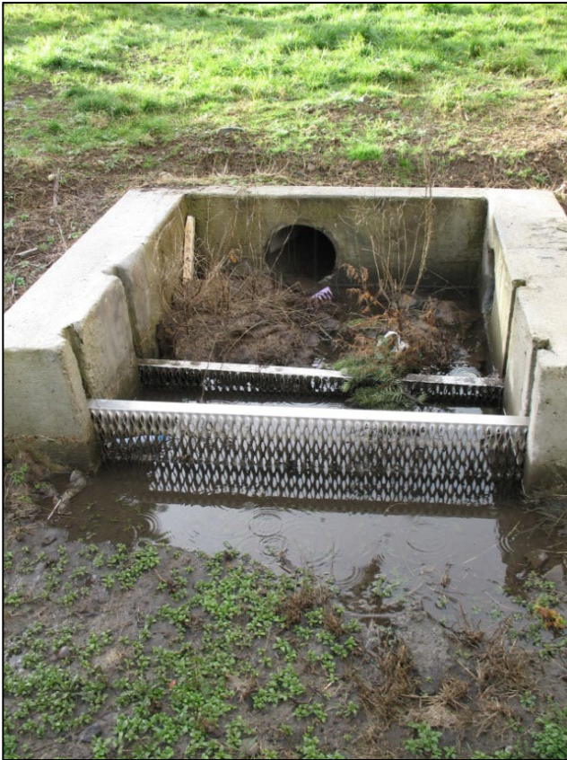
Sediment Trap with Accumulated Sediment
