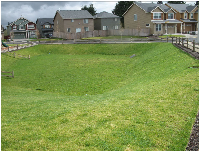
Example of a Manicured Detention Pond
