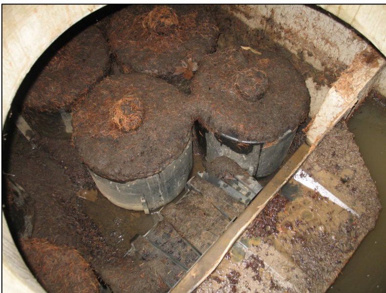
Media Cartridge Filter Vault with Accumulated Sediment
