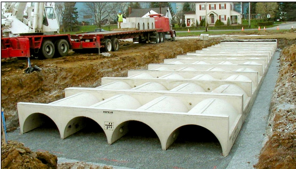
Example Proprietary Modular Detention System Installation
