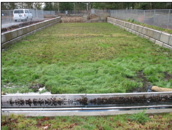
Example Typical Biofiltration Swale
