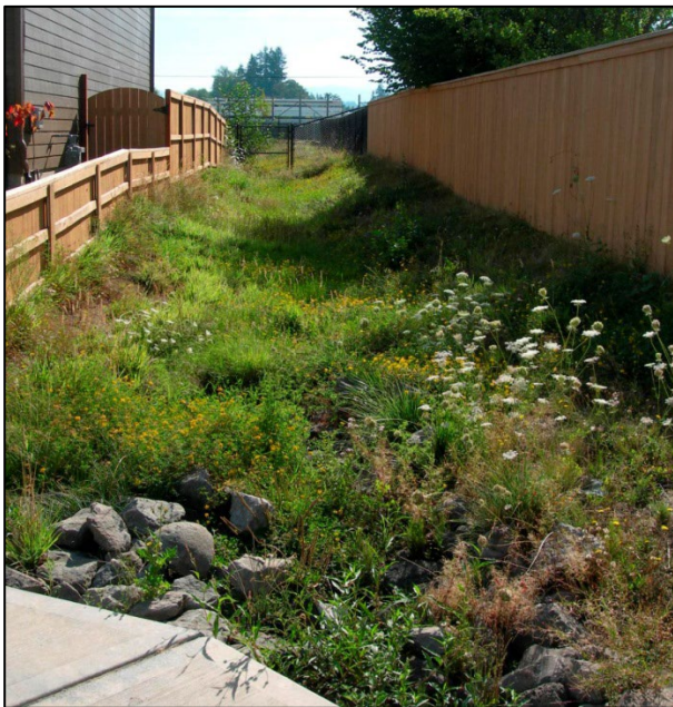
Example Typical Biofiltration Swale
