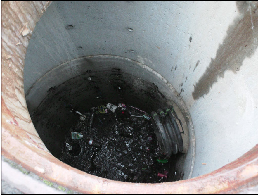
Drywell with Accumulated Trash
