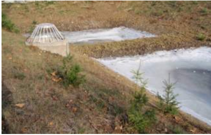
2-celled, deep water quality pond with cell dividing berm - cell 1 is on left for sediment collection
