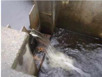
Weir is metal plate with a combination of a lower v-notch and upper, wide, rectangular notch
