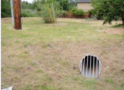
Aluminum horizontal debris barrier
