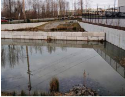
6' high black vinyl coated chain-link fence attached to inside face of concrete wall of water quality pond
