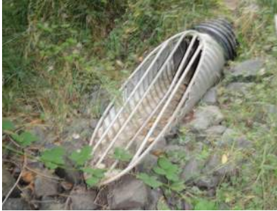
Aluminum horizontal debris barrier with bent bar needing repair
