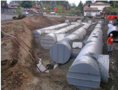
Looking at downstream end of a detention tank with end caps and connection pipe manifolds connected to adjacent detention pipes
