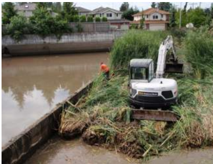
2-celled, deep water quality pond with concrete cell divider and perimeter walls. Non-routine maintenance of dredging and cattail removal shown.
