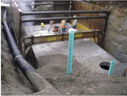
Detention vault installation (access hole and ventilation pipes visible)
