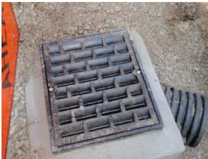
Type 1 catch basin with vaned grate
