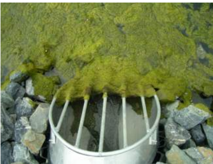
Aluminum horizontal debris barrier partially clogged with algae
