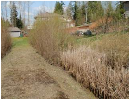
Before Maintenance: 2-celled, shallow water quality pond with cell dividing berm- cell 1 is on right of berm for sediment collection
