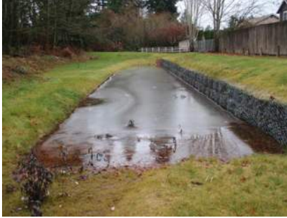
Pond with wall made of gabion basket (wire mesh rectangular baskets filled with rock)
