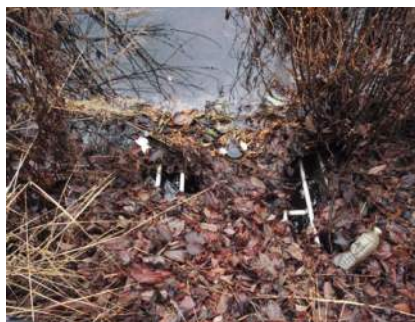
Aluminum horizontal debris barrier with bars covered with leaf and twig debris but water flowing below the barrier
