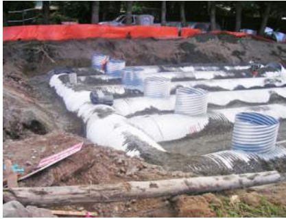
Detention tank with view of access risers
