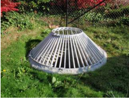
Stormwater pond Type 2 catch basin overflow structure with vertical conical galvanized steel debris barrier
