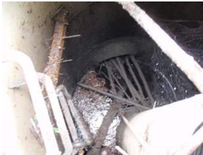
Type 2 catch basin stand-pipe flow control structure interior with debris- mostly tree limbs and fir needles
