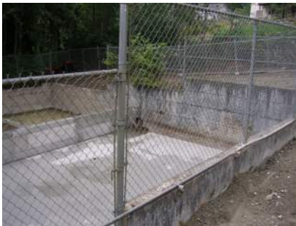
6' high galvanized chain-link fence with posts set in top of water quality pond perimeter wall
