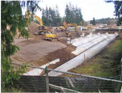
Detention tank in place and being covered up with compacted soil
