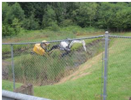
2-celled, water quality pond- cell for sediment collection is undergoing dredging for removal of sediment and cattail root mass
