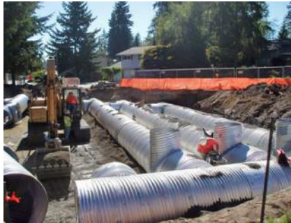
Looking at upstream end of detention tank connecting to pipe manifold (closest pipe in view running perpendicular to the rows of detention pipe)
