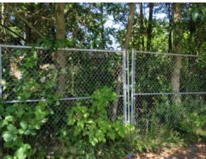
6' high x 8' wide galvanized chain-link double hung gate
