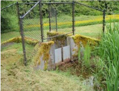
Weir is metal plate with deep, rectangular notch
