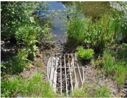
Aluminum horizontal debris barrier
