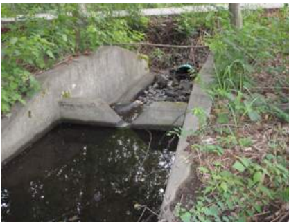
Weir is a v-notch in a concrete wall
