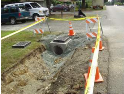
Type 1 catch basin with vaned grate
