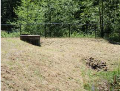
Typical location of a Type 2 catch basin with stand-pipe flow control structure for a stormwater pond
