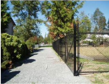
6' high black vinyl coated chain-link fence along perimeter of a detention pond
