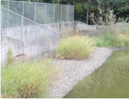
6' high galvanized chain-link fence with posts set in top of water quality pond access road wall
