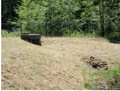
Pond berm with Type 2 Catch Basin flow control structure at top of berm
