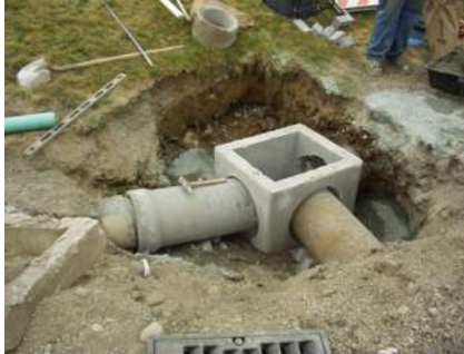
Type 1 catch basin connecting concrete pipe
