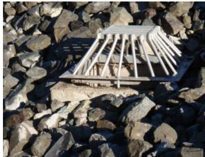
Stormwater pond with Type 1 catch basin with galvanized steel, bee-hive debris barrier
