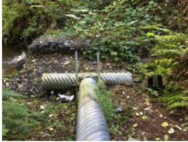
Example of slope drain diffuser tee
