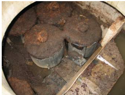
Media Cartridge Filter Vault with Accumulated Sediment
