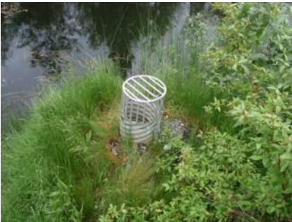
Stormwater pond overflow structure with vertical top-hat aluminum debris barrier set in pea-gravel filtration cone
