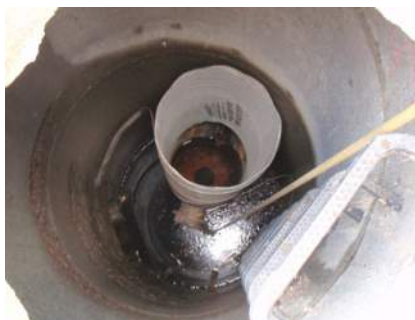
Hole in disk at bottom of standpipe is a flow regulating orifice
