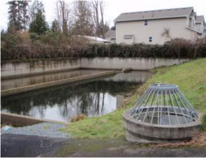
2-celled, deep water quality pond with concrete cell divider and perimeter walls- cell 1 in the front is for sediment collection
