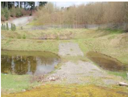
2-celled, deep water quality pond cell 1 in the back is for sediment collection cell 2 in front has access road to cell 1 running through it and over the cell dividing berm
