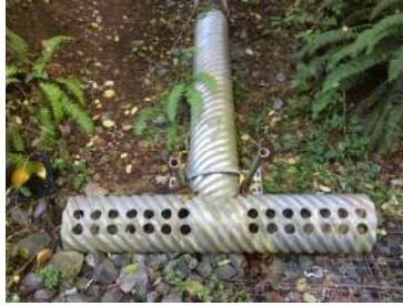
Example of slope drain diffuser tee
