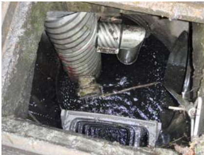
View from rectangular access hole showing the access ladder and standpipe with orifice elbow and shear gate with attached lift rod
