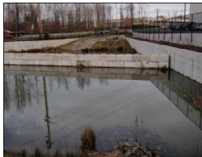
2-celled, deep water quality pond with concrete perimeter walls and ecology block cell divider
