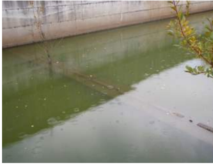
Close-up of submerged concrete block (known as "ecology block") cell divider wall
