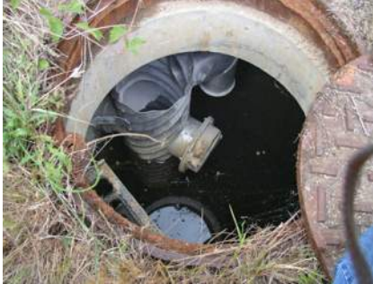
View from open round access hole showing the standpipe with orifice elbow and shear gate with its lift rod detached
