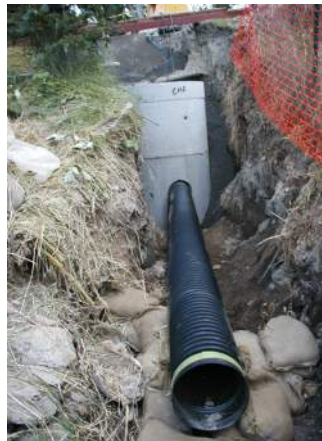
Type 2 catch basin connecting plastic pipe
