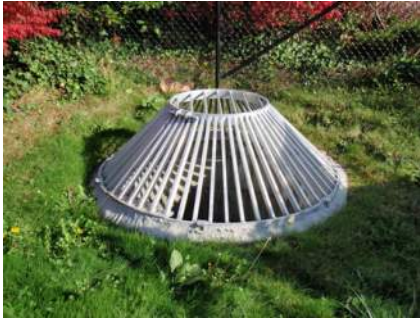
Stormwater pond Type 2 catch basin overflow structure with vertical conical debris barrier
