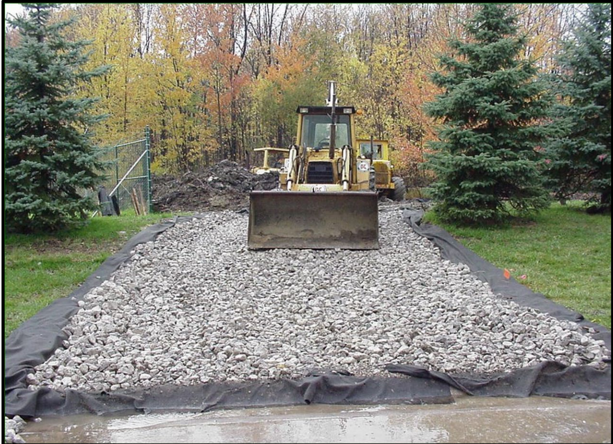
Figure 6. Stabilized Construction Access.
