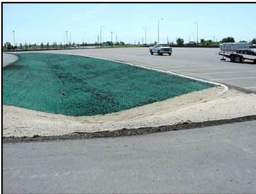
Figure 1. Hydroseeding Method.
