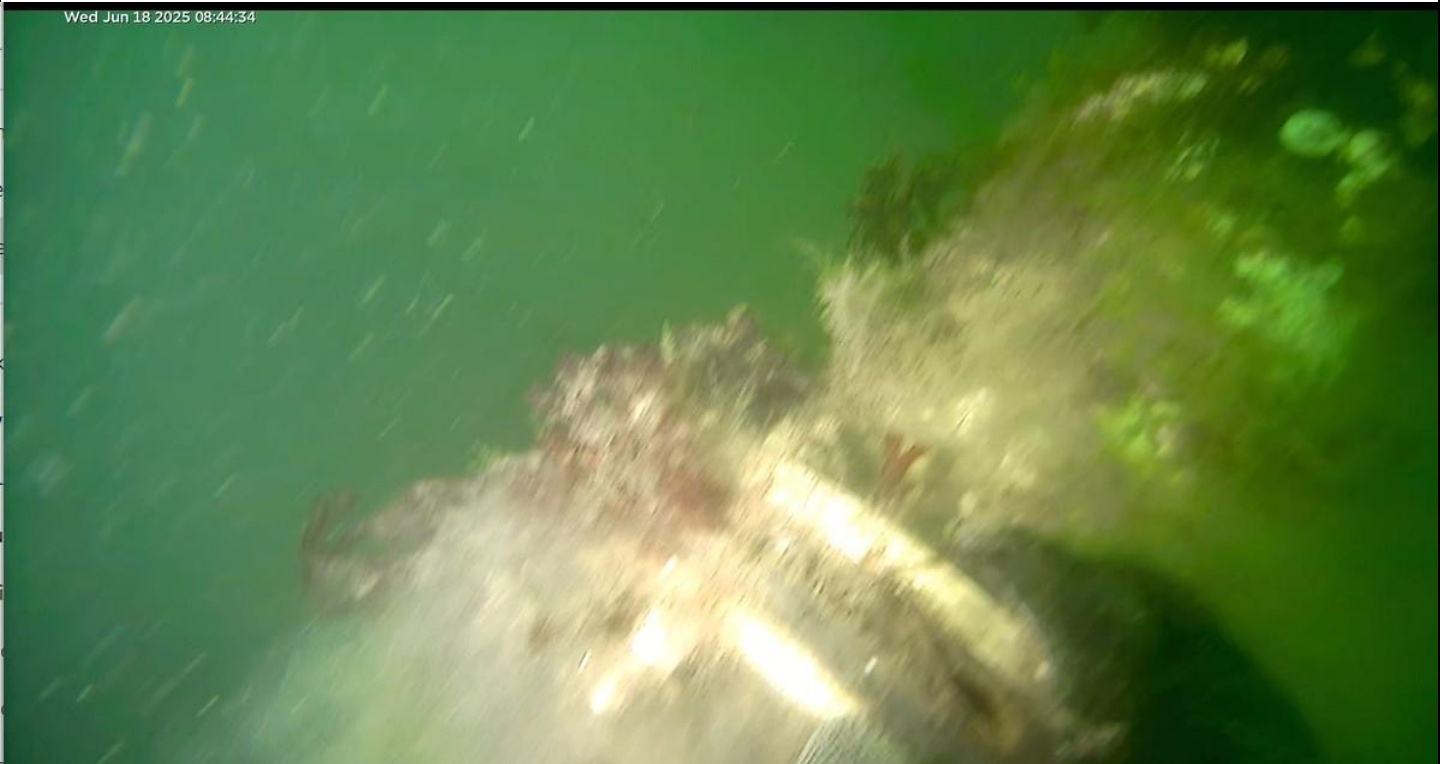
Photo #5: Flange Duckbill to Riser
