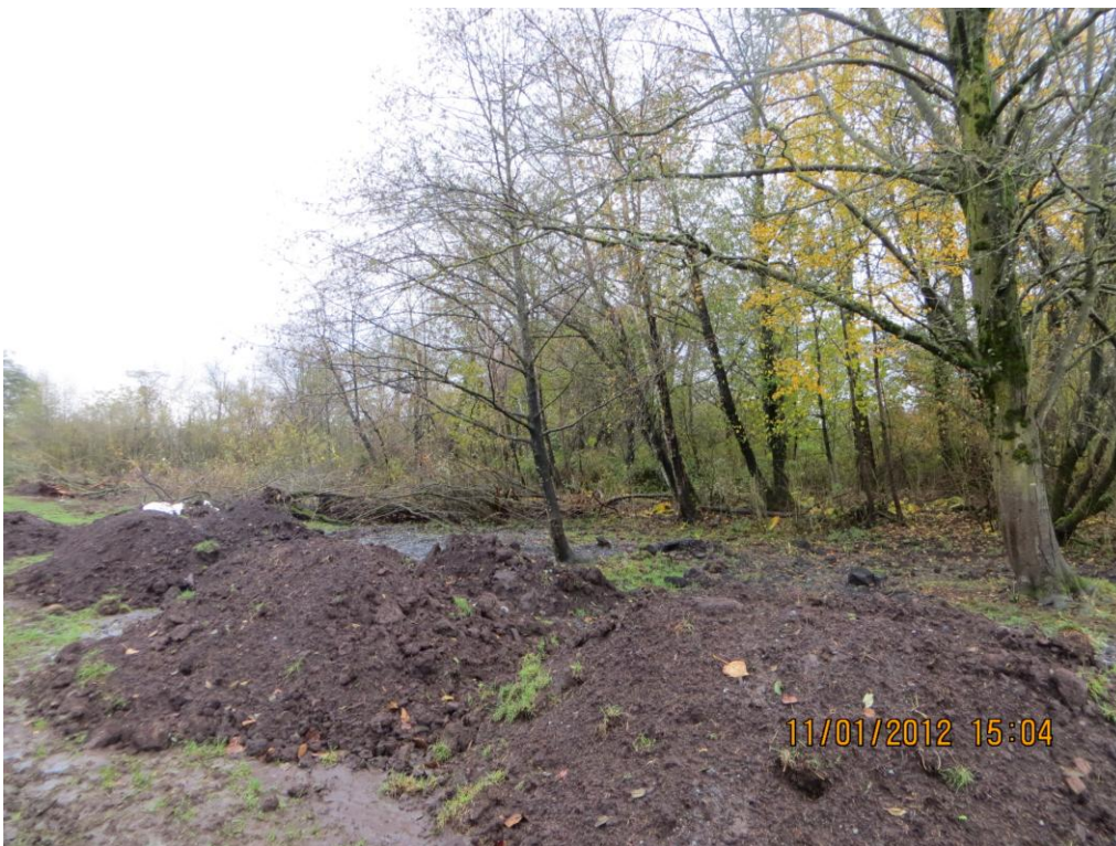
Photo 4: Piles of excavated soils placed in wetlands on east side of Squaw Creek. Constitutes violation of RCW 90.48. Mr. Crabtree has agreed to halt all excavation work and install a silt fence between these soil piles and the wetlands to reduce the risk of sediment entering the wetlands and Squaw Creek.
