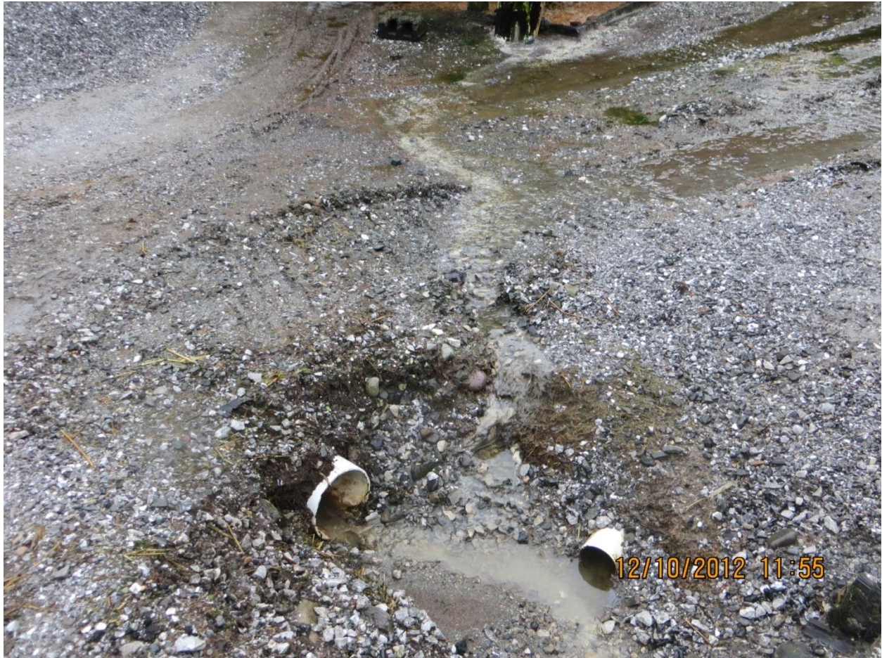
Photo 8: Depicts contaminated leachate trail flowing into pipes that flow convey flow to the South Cornell Creek Road ditch (state waters). Smaller pipe in right field of photo is of unknown origin and needs to be tested.
