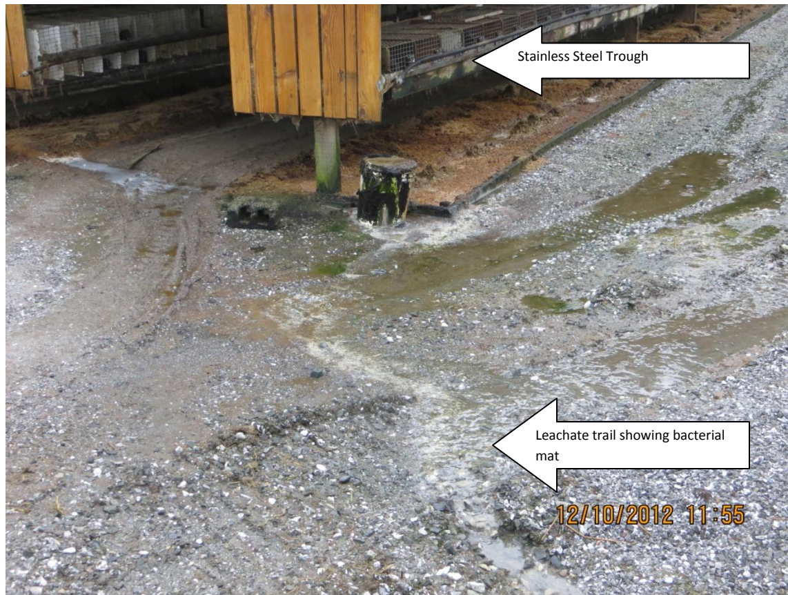
Photo 6: Same bucket depicted in photo 2 showing stainless steel watering trough and bucket overflowing with mink food waste contaminated with manure. Additionally, note the leachate trail flowing toward piping that conveys the contamination to the south Cornell Creek Road ditch.
