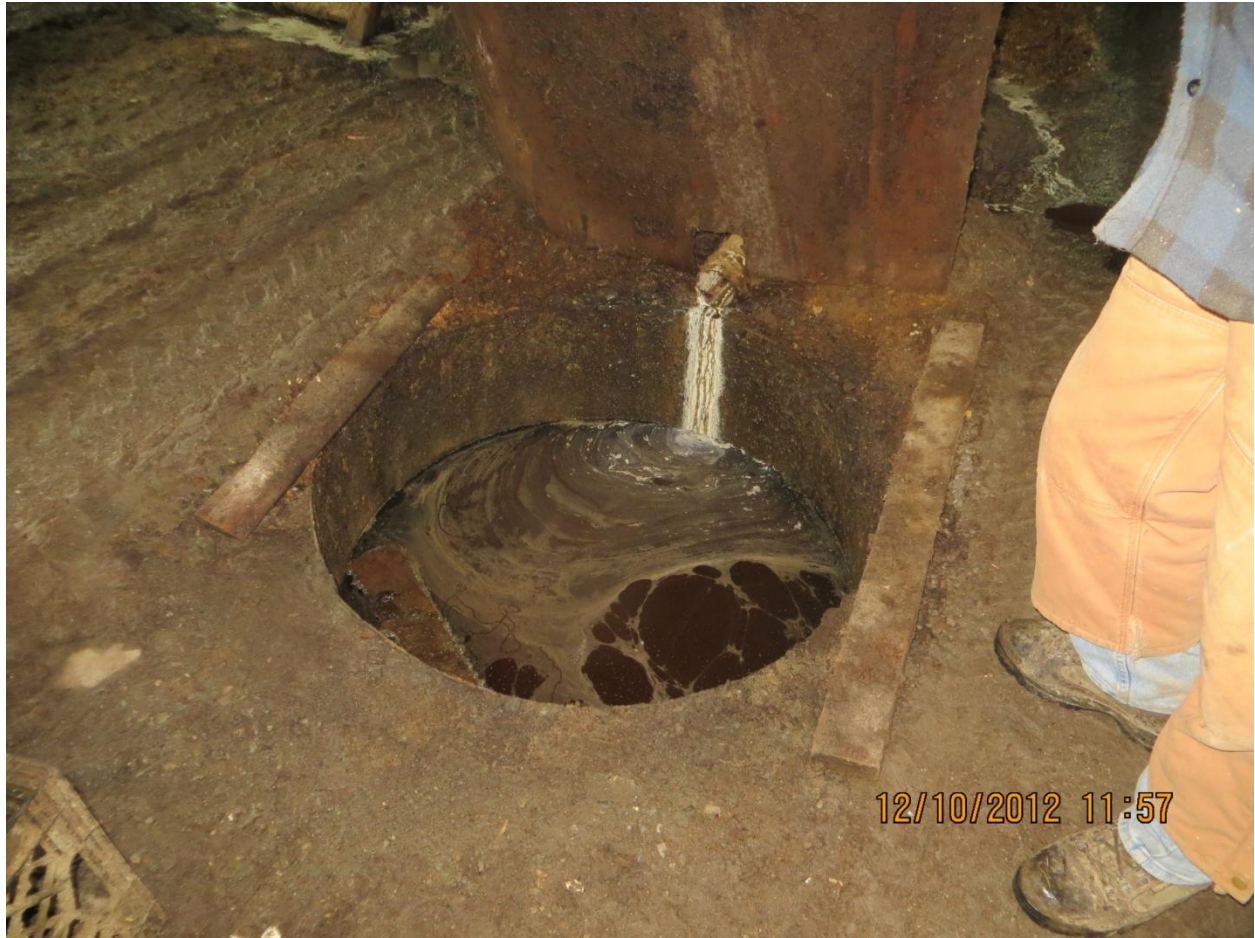
Photo 14: Shows leachate collection system Mr. Marr had installed in two of his barns. This was marginally functional, but Mr. Marr stated that he could not afford to install this in all of his mink barns.
