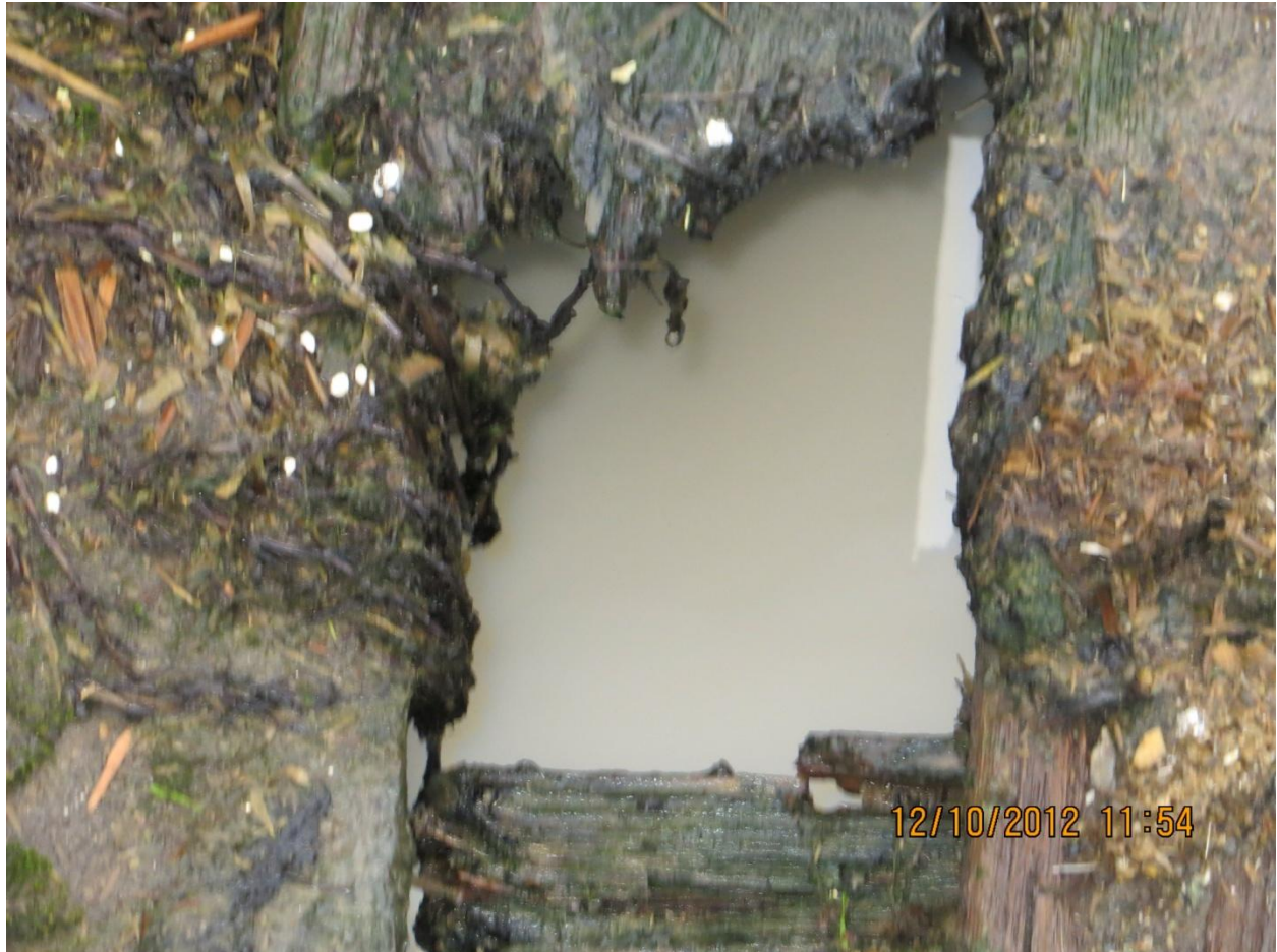
Photo 10: Photo showing “milk colored” water depicted in Photo 10. Sample collected from this sump which was analyzed for fecal coliform bacteria came back from the laboratory at 120,000 CFUs per 100 ml water. The state standard is 200 CFUs per 100ml water. Mr. Marr admitted later that his kitchen sink was plumbed into this sump. When we returned on January 7, 2013, Mr. Marr stated that the sink had been disconnected from this sump and was no longer contributing to the contaminated discharges. The sample collected on January 7, 2013 came back from the lab at 2,400CFUs per 100 ml water showing a vast reduction.
