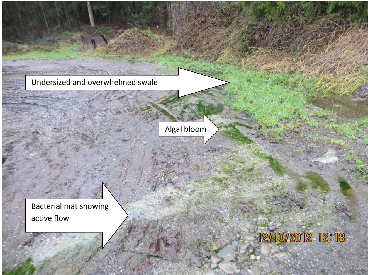
Photo 16: Photo shows bacterial mat flowing with active flow from the area depicted in Photo 16. Note the vastly undersized an overwhelmed vegetated swale and more of the blue-green algal bloom.
