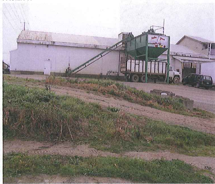
PHOTO #:08 DATE: 10/24/13 TAKEN BY: JEANNE TRAN DESCRIPTION: SCREENED SOLIDS ARE CONVEYED OUT OF THE PLANT AND INTO TRUCKS TO BE TAKEN BACK TO THE FIELD.
