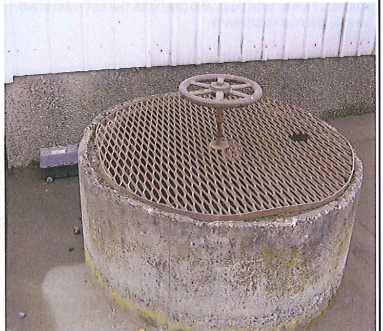
PHOTO #:010 DATE: 10/24/13 TAKEN BY: JEANNE TRAN DESCRIPTION: SOME AREAS OF THE PLANT ARE NOT PAVED, AND STORMWATER RUNOFF DRAINS INTO UNDERGROUND SUMPS, WHICH DRAIN INTO AN UNDERGROUND COLLECTION SUMP BEFORE IT IS GRAVITY DRAINED TO THE SETTLING POND.
