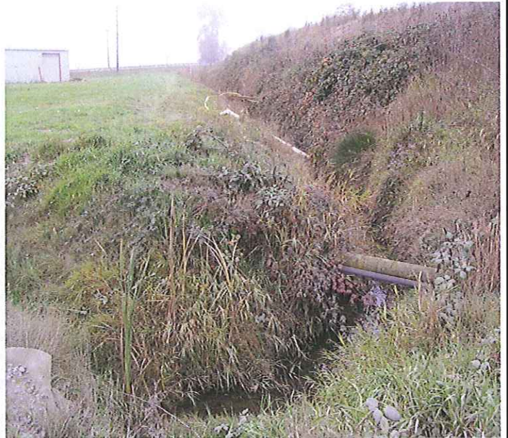
PHOTO #14 DATE: 10/24/13 TAKEN BY: JEANNE TRAN DESCRIPTION: CURRENTLY, THE SETTLING POND'S OUTLET IS PIPED UNDER THE ROADS TO THE LAND APPLICATION FIELD FOR IRRIGATION.
