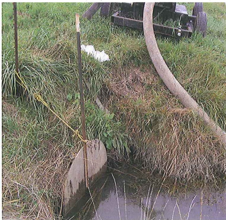
PHOTO #:21 DATE: 10/24/13 TAKEN BY: JEANNE TRAN DESCRIPTION: EACH END OF THE DITCH IS BLOCKED OFF WITH A WOODEN PLATE TO PREVENT FLOW FROM DRAINING OFF SITE.
