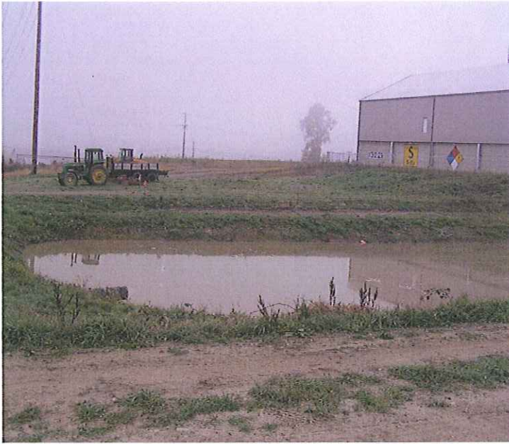
PHOTO #13 DATE: 10/24/13 TAKEN BY: JEANNE TRAN DESCRIPTION: THE SETTLING POND THAT HUGHES FARMS SHARES WITH NEIGHBORING FACILITY, CHEMTRADE SULEX. SINCE HUGHES FARMS DISCHARGES INTO THIS SETTLING POND ON A REGULAR BASIS IN COMPARISON TO CHEMTRADE SULEX, HUGHES FARMS MAINTAINS AND DREDGES THE SETTLING POND WHENEVER IT IS NECESSARY.
