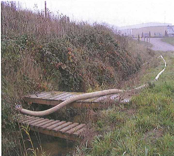
PHOTO #15 DATE: 10/24/13 TAKEN BY: JEANNE TRAN DESCRIPTION: A CLOSE UP VIEW OF THE POND'S OUTLET BEING PIPED ACROSS AND UNDER THE FACILITY ACCESS ROAD, THEN TRAVELS WEST ACROSS AND UNDERNEATH FARM TO MARKET ROAD TO THE LAND APPLICATION SITE.
