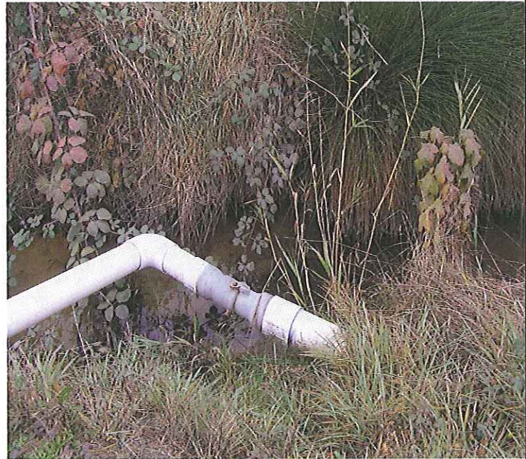
PHOTO #16 DATE: 10/24/13 TAKEN BY: JEANNE TRAN DESCRIPTION: AFTER CROSSING THE FACILITY'S ACCESS ROAD, THE PIPE IS ELBOWED AND CONTINUES UNDERGROUND AND ACROSS THE FARM TO MARKET ROAD TO THE LAND APPLICATION SITE.
