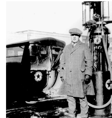
Photographs of the original gasoline pumps at the Rosalia site; a cleanup site under the Clean Sites Initiative
