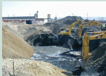
Trac-boes excavating in 'pit' area where pesticides were originally dumped.
