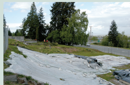
Former smelter site along East Marine View Drive showing lots where houses used to be.
