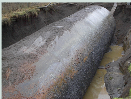
30,000 gallon underground storage tank (photo courtesy of Dom Reale)
