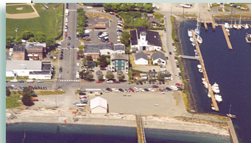
Ariel view after site cleanup (Photo courtesy of Darryl Swenson)
