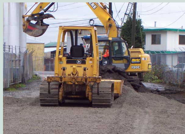
South Park Soil Remediation Project (photo courtesy of Seattle Public Utilities)
