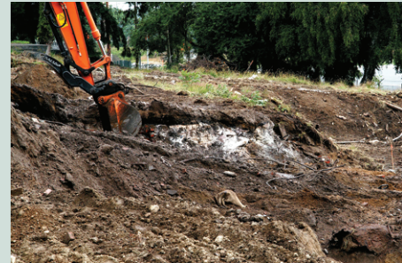
Cleanup of arsenic trioxide product (white material). This material was about 40% arsenic.
