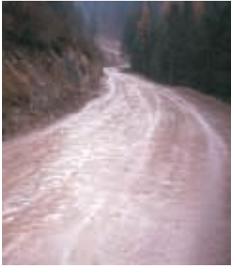
Before: Water on the road delivers sediment to the creek.
