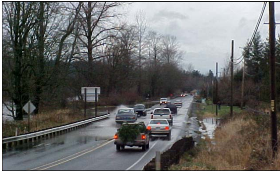
Figure 5. Stormwater runoff flowing off roadway during a 2005 January winter storm.
