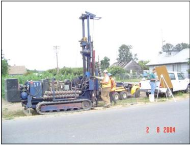
Track-mounted hollow stem auger drill rig in operation
