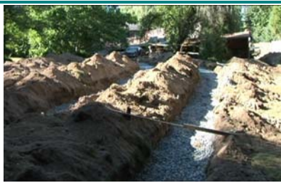
The new drainfield
