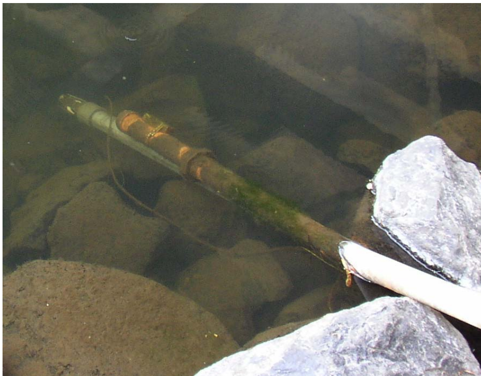
Figure 3. In-pipe sonde deployment.
