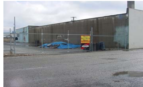
Parking area on North side of Building
