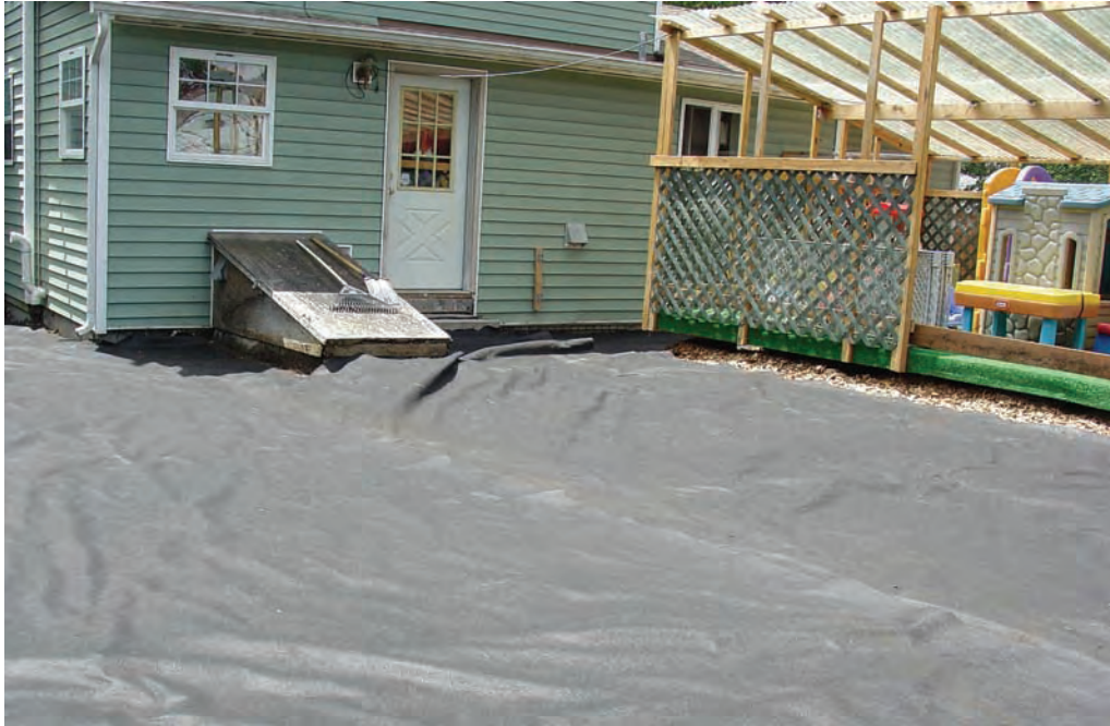
Image 10a. Geotextile barrier placed over soil
