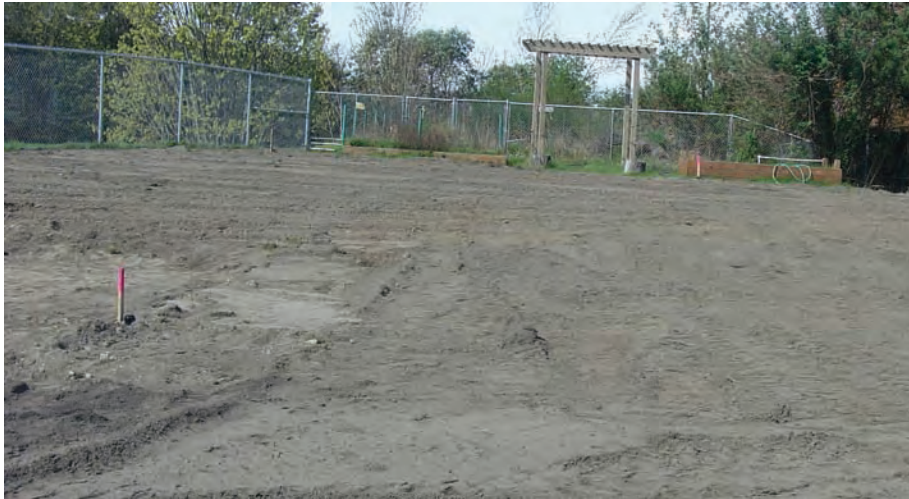
Image 4. Mixing contaminated soil with clean soil
