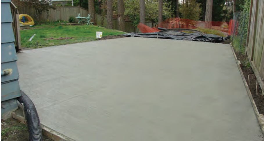
Image 3. Covering contaminated soil with concrete
