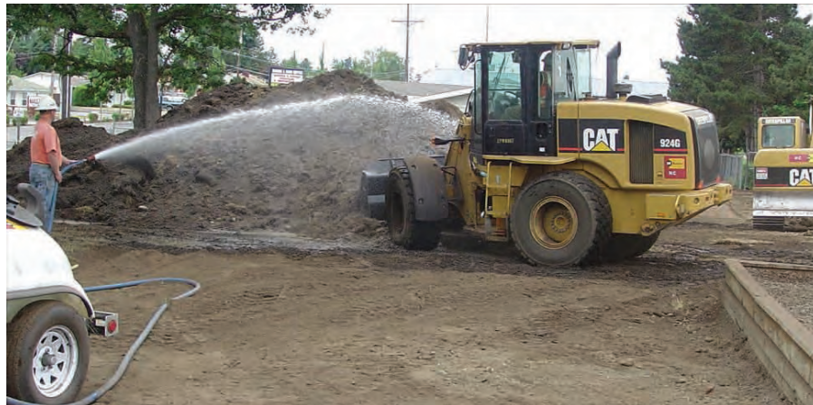
Image 8b. Soil removal and watering to control dust
