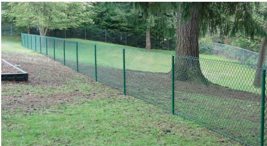
Image 5. Fencing off area with contaminated soil
