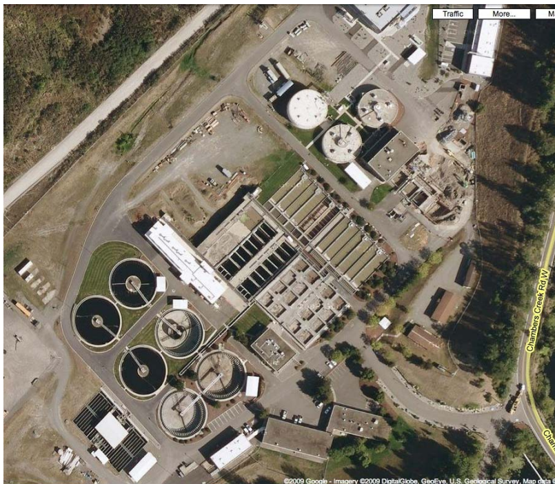
Figure C-5. Aerial photo of the Chambers Creek Wastewater Treatment Plant.
