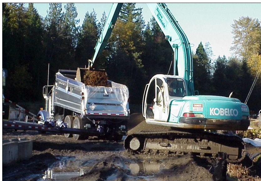
Excavation of petroleum contaminated soils for off-site disposal.
