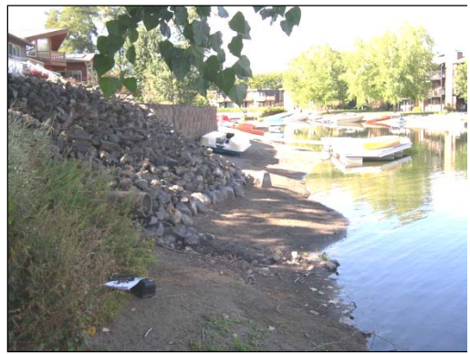
One of two newly discovered outfalls to Liberty Lake.
