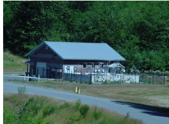
FTA Waste Water Treatment Facility
