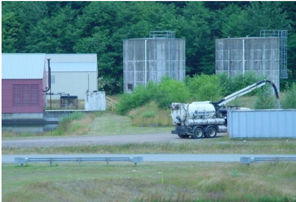
Vacuum truck cleaning FTA drains
