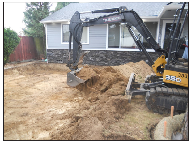
Contractors remove contaminated soil on yard.
