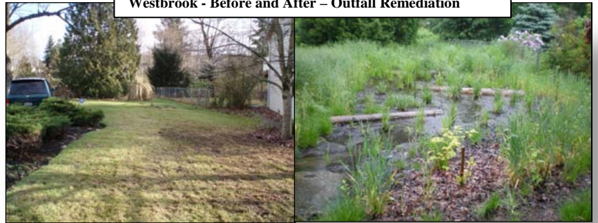
Westbrook - Before and After – Outfall Remediation
