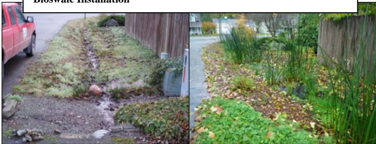
North Creek Park Division 1 Subdivision – Before and After – Bioswale Installation
