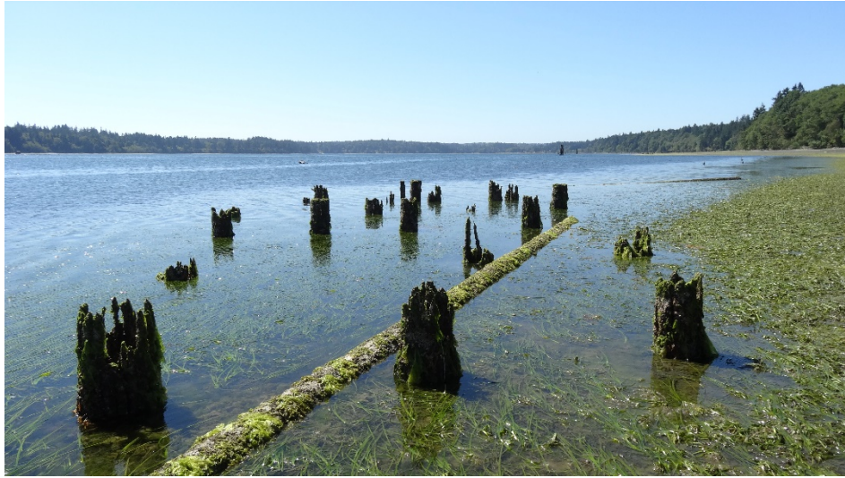
Figure 16-6. Decayed piling stubs in eelgrass at the former Port Gamble sawmill in Port Gamble, WA. Additional care was taken to hand excavate around individual pilings so they could be removed, which minimized disturbance to the eelgrass bed.
