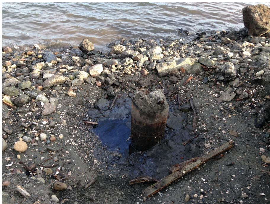
Figure 16-5. Partially excavated piling stub on intertidal beach at the former Port Gamble sawmill in Port Gamble, WA. A vibratory hammer later facilitated full extraction of this stub. Visible sheen on water's surface is creosote leaching into the surrounding environment.
