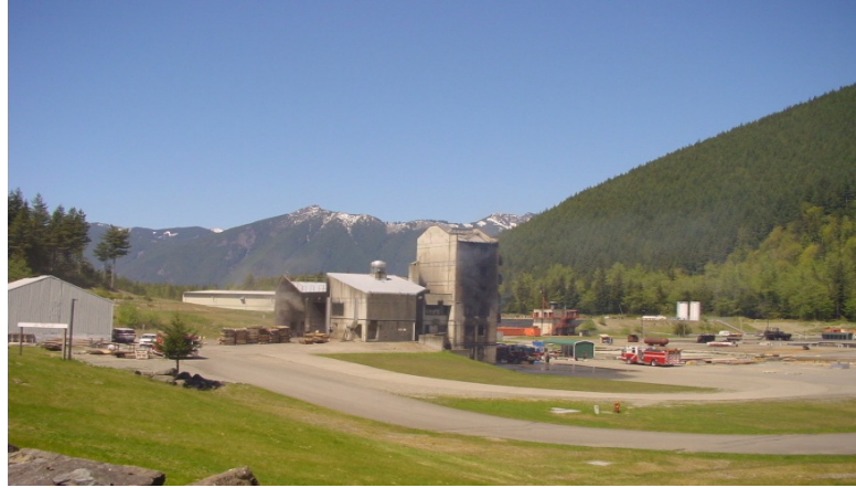
The Fire Training Academy training grounds.
