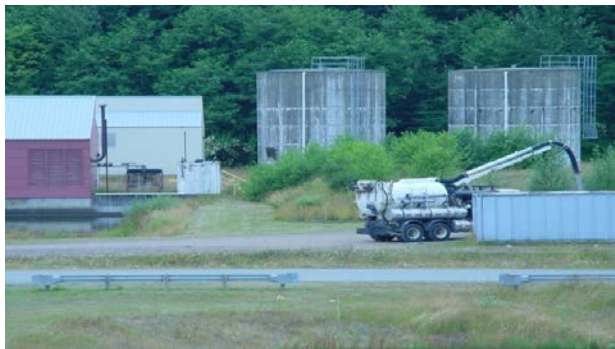
Vacuum truck cleaning Fire Training Academy drains.
