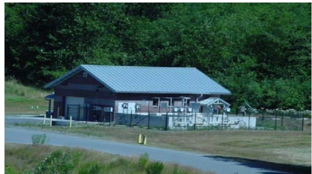
The Fire Training Academy waste water treatment facility.
