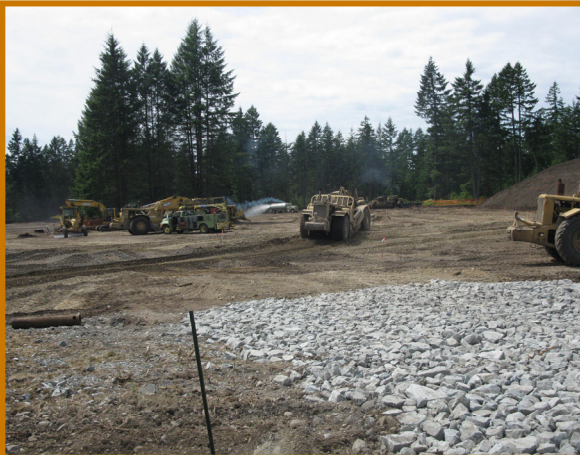
Creekside Village development site
