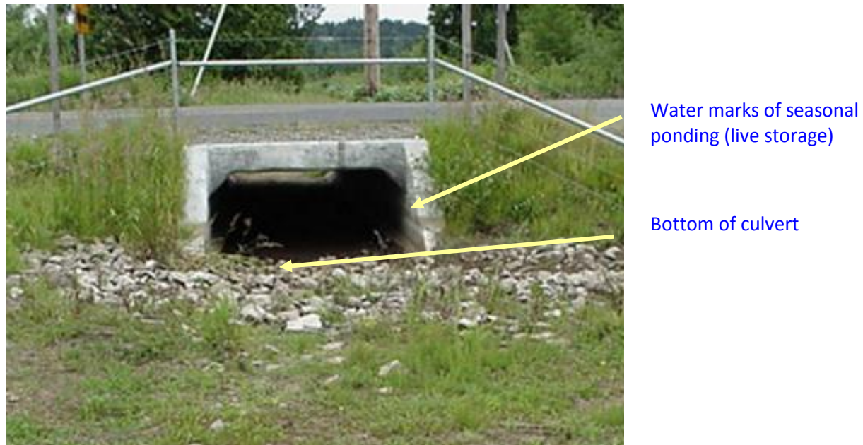
Figure 24. A box culvert that is the outlet of a Depressional wetland. The live storage is measured as the distance between the bottom of the culvert and the water marks on the side. The distance here is approximately 15 in.
