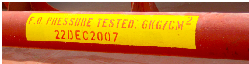
Fuel oil line marked with pressure test date.
