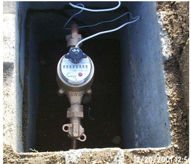
Figure 9.1 Water treatment systems for contaminated public wells and connecting affected homeowners to a public water supply are examples of uses of Safe Drinking Water Grants
