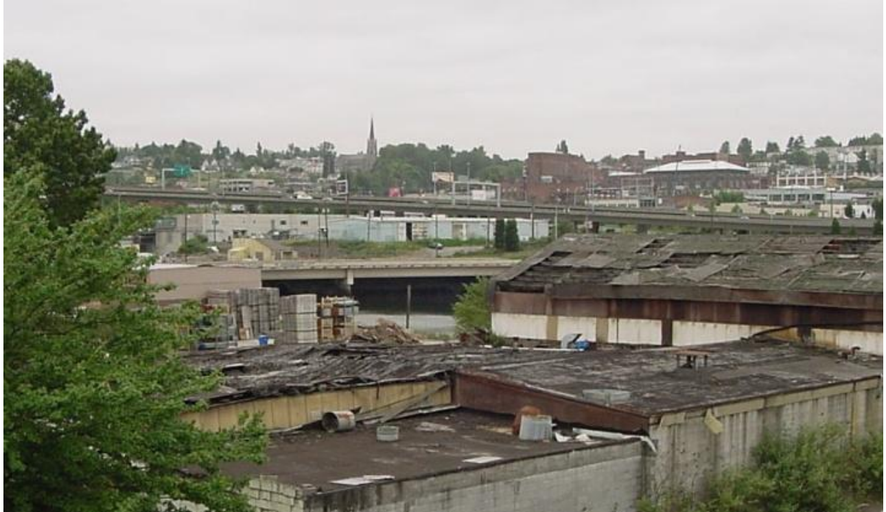
Figure 6.1 Thea Foss Waterway Tacoma – Pre cleanup
