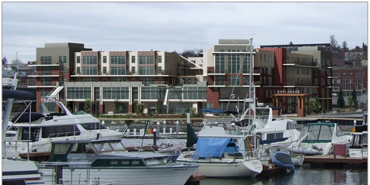
Figure 6.2 Thea Foss Waterway Tacoma – Post Cleanup with Development Underway
