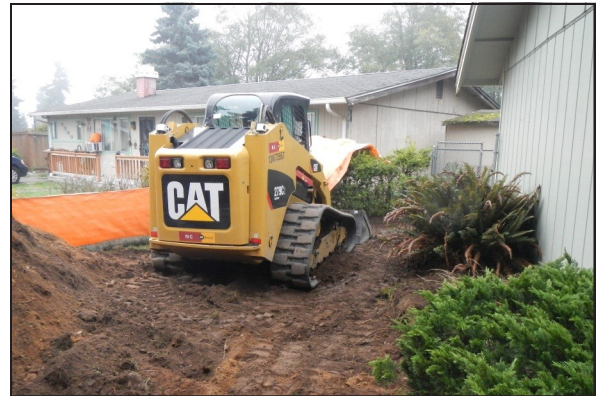
We remove the top 12 to 18 inches of contaminated soil.
