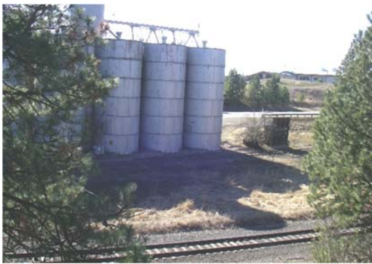
Looking South at the Grain Handling Facility
