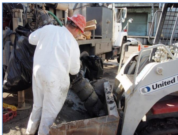
Photo 11: Worker installing a new remedial well at the former Lilyblad property.
