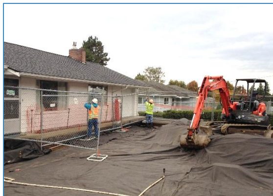
Photo 2: Contractors put up protective fencing in a yard in Everett
