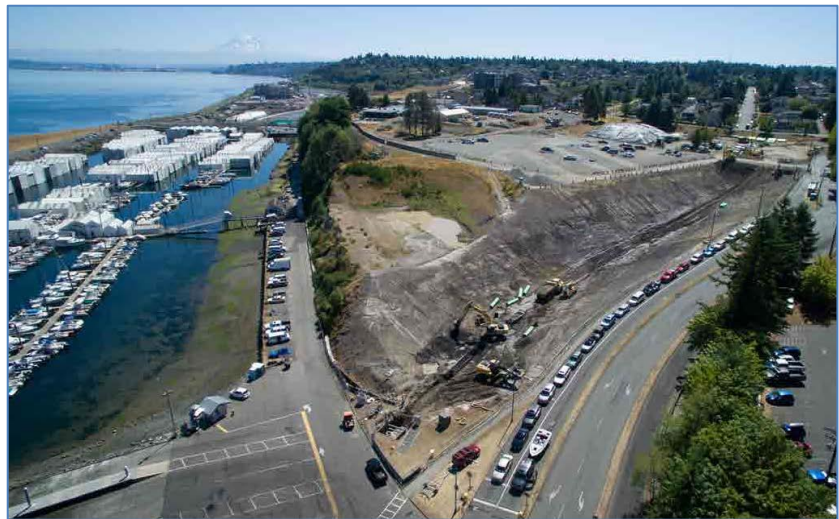
Photo 5: Point Defiance Trails Project during construction
