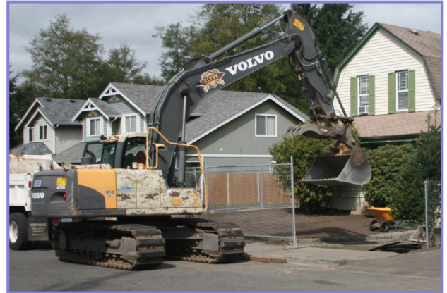
Contractors excavate contaminated soil from a yard in Tacoma.
