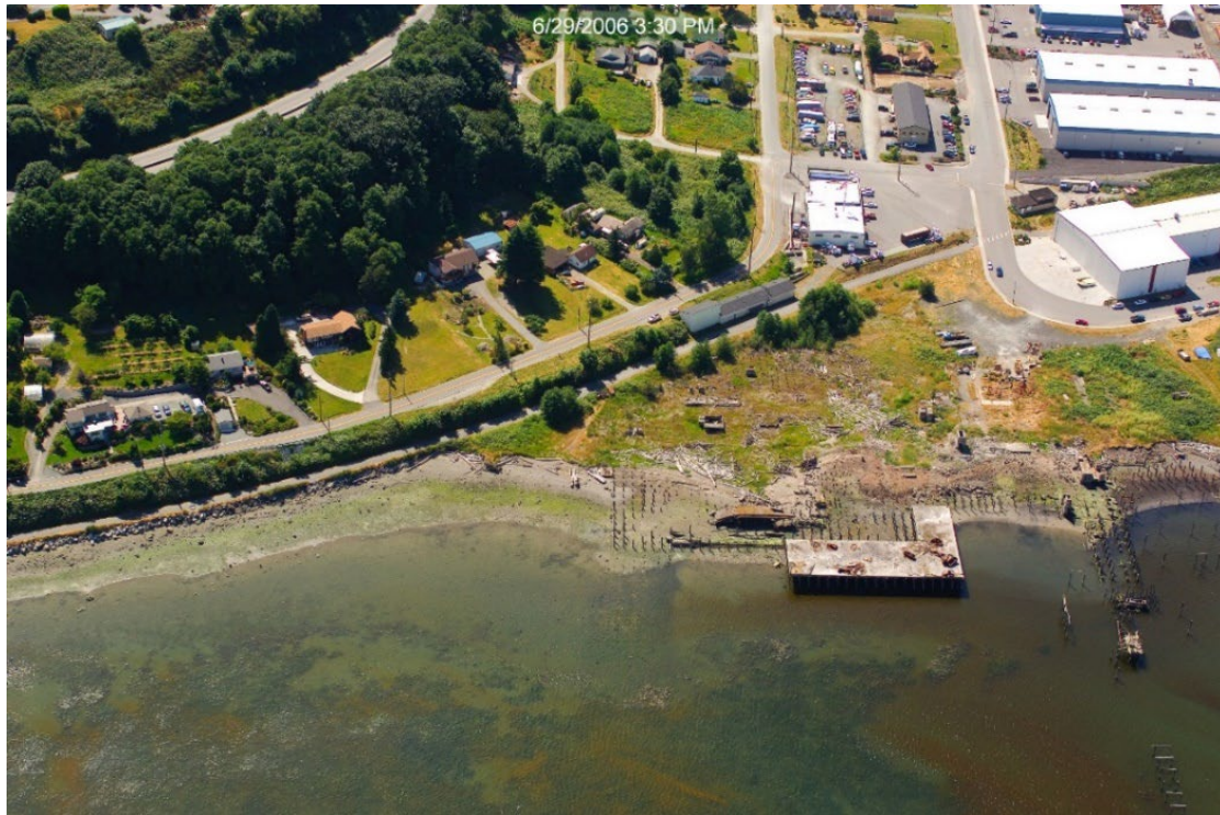
Figure 32: Custom Plywood site before cleanup construction.
