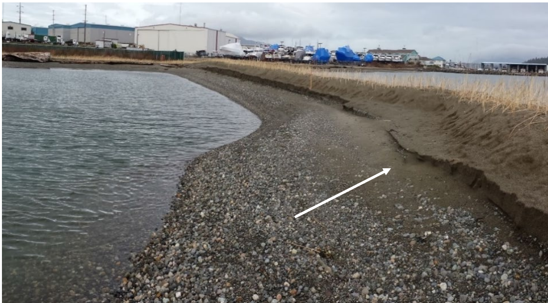
Figure 35: Custom Plywood site with erosion of the wetland bank during a storm event.
