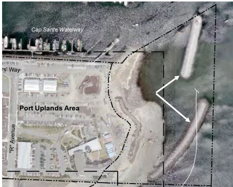
Figure 30: Scott Paper Mill site wave attenuation structures.
