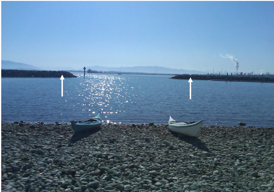
Figure 29: Scott Paper Mill after cleanup construction showing structures to attenuate waves and lessen impacts of 100-year storms (as currently defined by FEMA) projected to occur every 25 years.
