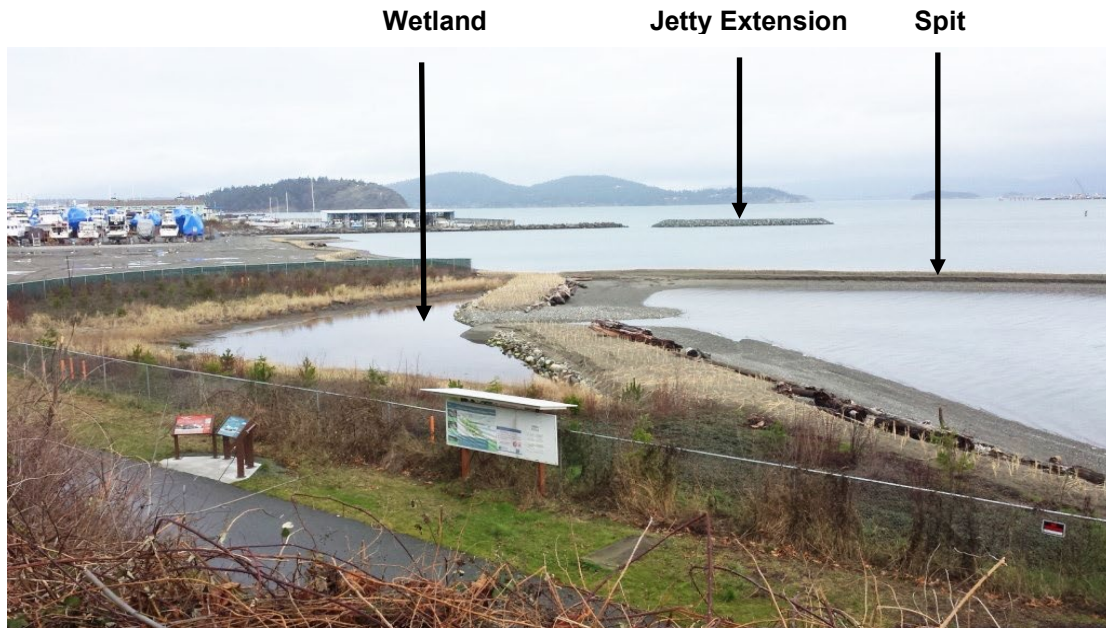
Figure 33: Custom Plywood site after cleanup construction.
