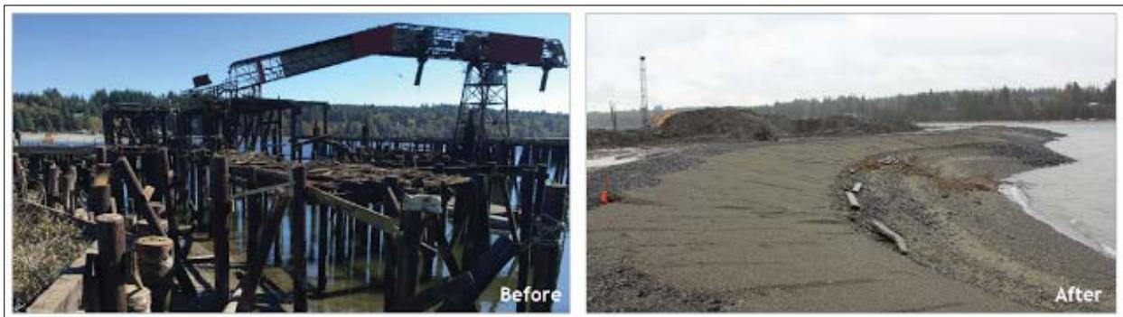
**Photo 17a and b:** More than 8,500 creosote-soaked pilings and 5,600 tons of steel, concrete, and debris were removed from the Port Gamble Bay and Mill cleanup site between 2015 and 2017. As of 2017, shellfish and wildlife are returning to where the sawmill once stood. Photo credit: Ecology (2015, 2017)
