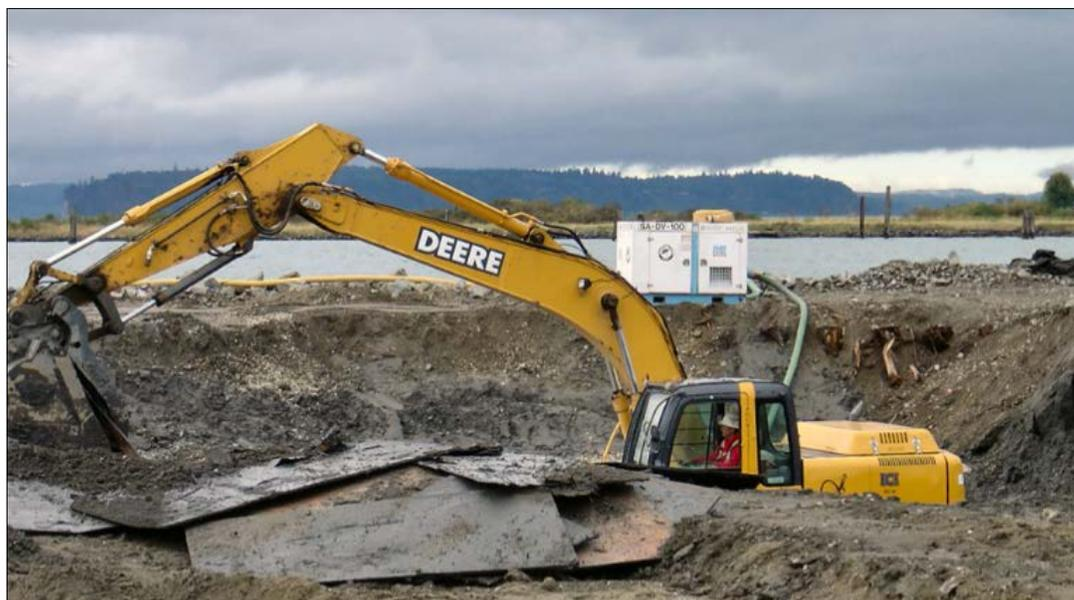
**Photo 37:** Deep-soil excavation helped clean up groundwater impacted by petroleum contamination at the West End site on Everett's waterfront. Photo credit: Ecology (2007).
