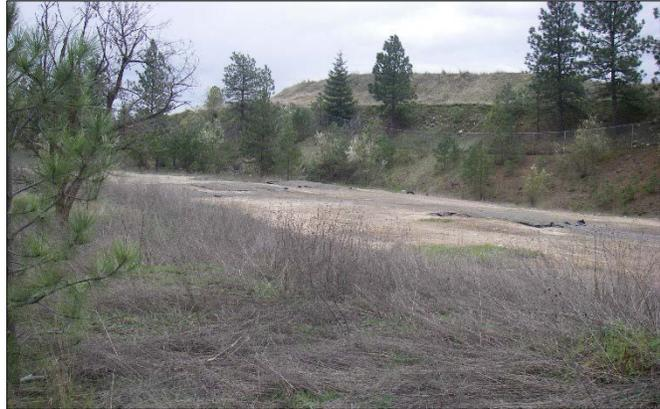
The cleanup remedy for the Holcim Inc. site was constructed from July through November 2016. The CKD deposit near the Spokane River (regraded area in foreground of bottom photo) was excavated and combined with the other CKD deposit further away from the river (the reseeded, sloped area on hill in photo).
