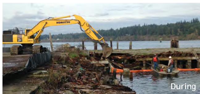
Top: Removal of key sources of contamination - creosote piles and wood waste - from the mill area.
